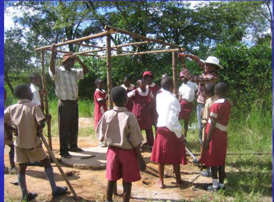
*Mounting and linking the upright poles and roof timbers with wire.*
