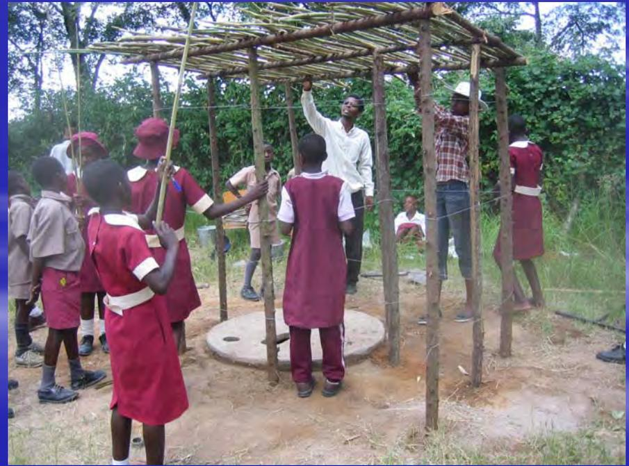
***Adding a plastic sheet over the reeds of the roof and grass to the walls.
