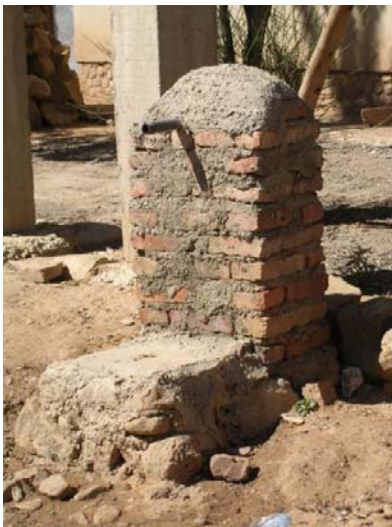
Figure 5-14. Tap stands are small brick columns built around a water pipe.
