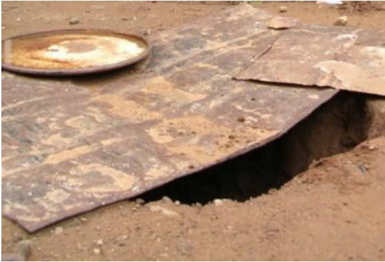
Figure 5-11. Wastewater is disposed of in unsealed dumping holes. Here, the hole is located inside a housing compound.
