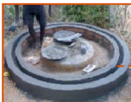
Figure 3.6: Channels during and after construction
