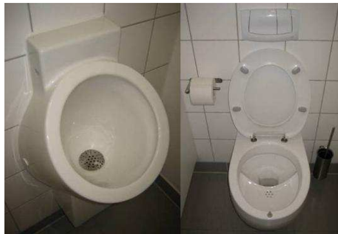
Fig. 4: Left: waterless urinal (Keramag). Right: urine-diversion flush toilet (Roediger) at GTZ main building; note the two buttons for flushing: the small one is for the urine flush, the larger one for the faeces flush (source: L. Ulrich, January 2009).
