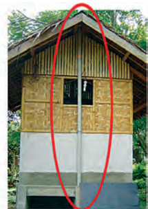
DIAMETER TOO SMALL
