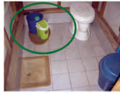
COVER MATERIAL & WASTE BIN FOR DISPOSAL OF TOILET PAPER
