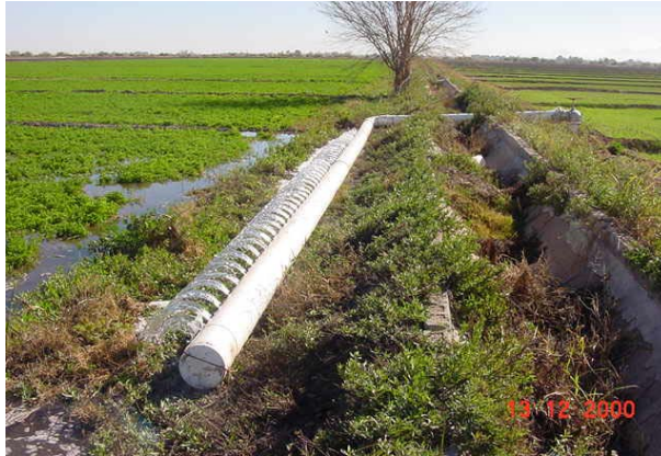
Figure 3.11. Plastic gated pipe for furrow irrigation (From Dr. G. P. Merkley personal collection).
