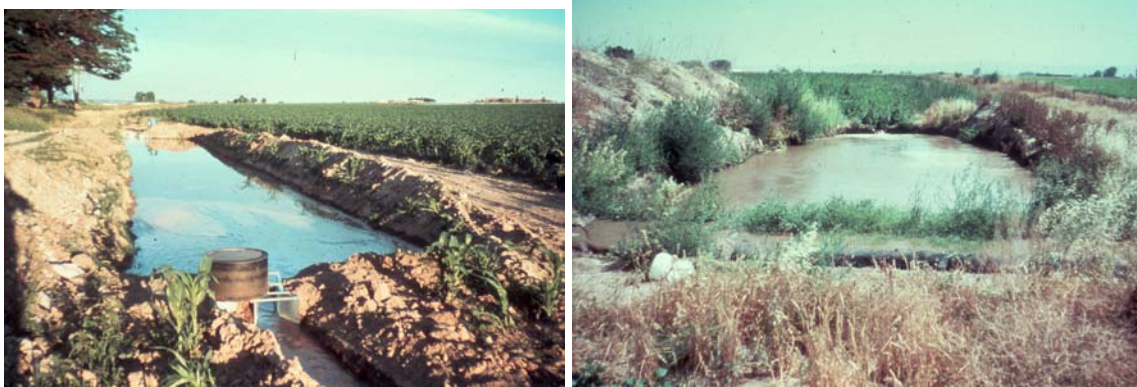
Fig. 3.6. Two views of typical tailwater recovery and reuse facilities.
