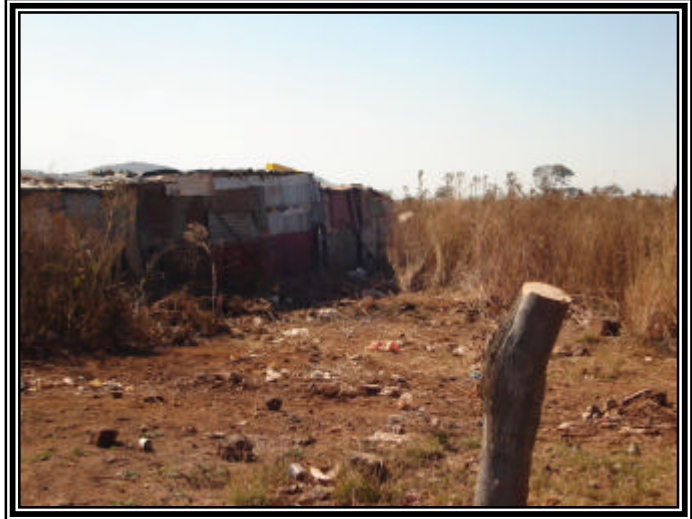
Houses at the boundary of Itereleng with no fire break to protect it.
