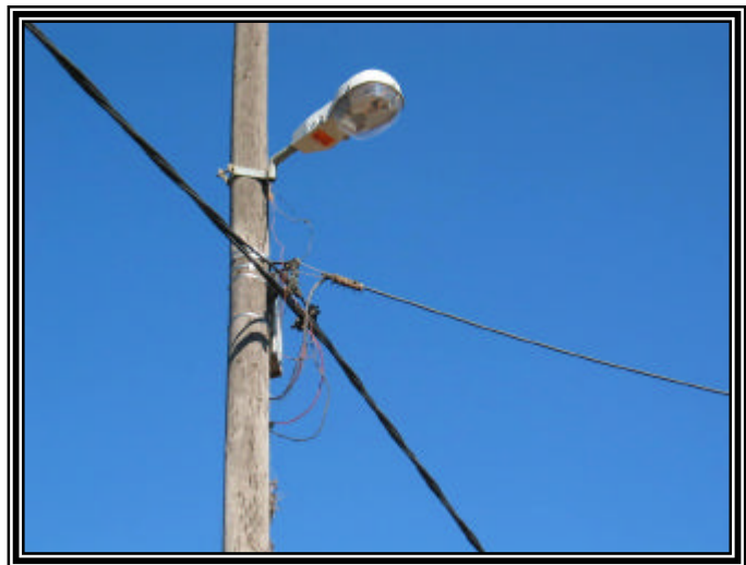
Residents do their own electrical connections. (People doing things for themselves)
