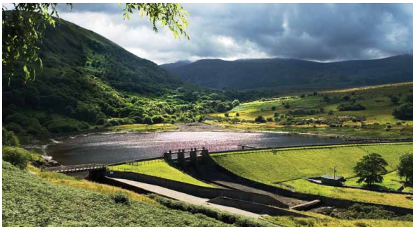
Coedty dam and reservoir, Wales
