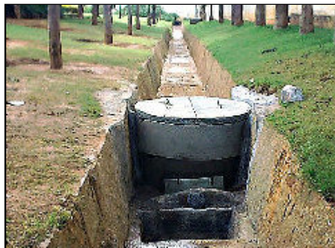
USEFUL DEVICE: A water recharge well
