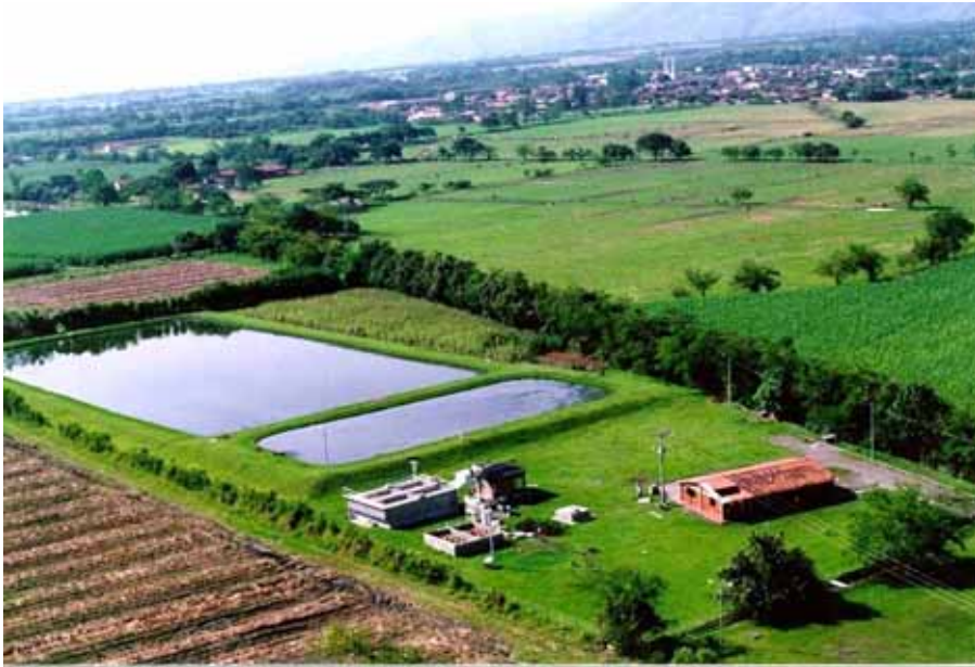
Figure 2. WSP system at Ginebra in southwest Colombia (population 9,000; wastewater flow 27 l/s) comprising an anaerobic pond and a facultative pond. The WSP effluent is used for the irrigation of sugar cane.
