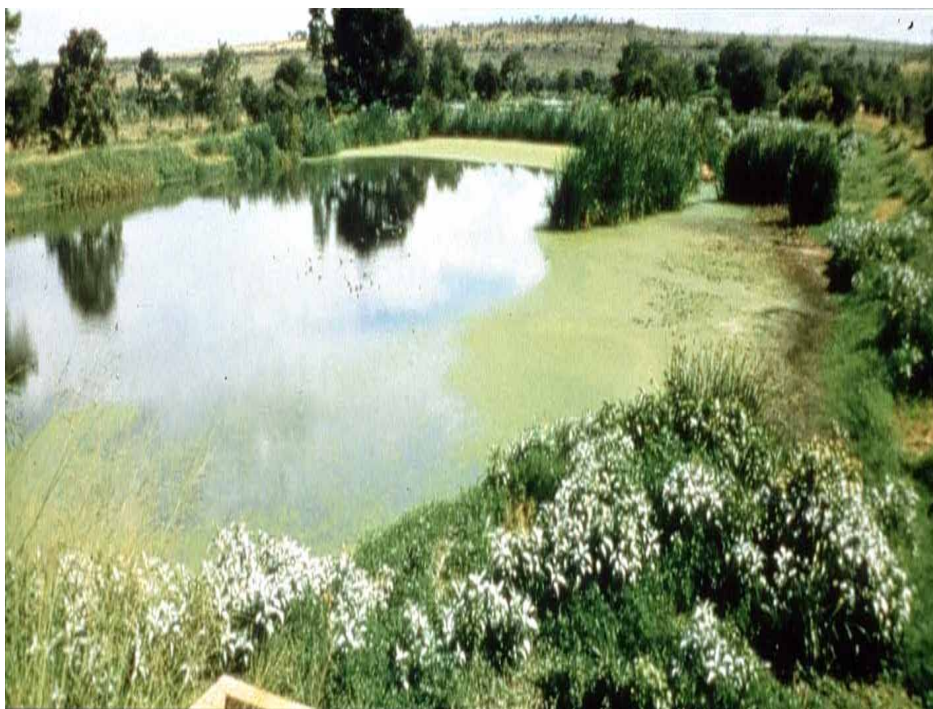
Figure 16. An example of a WSP system suffering from total maintenance neglect.
