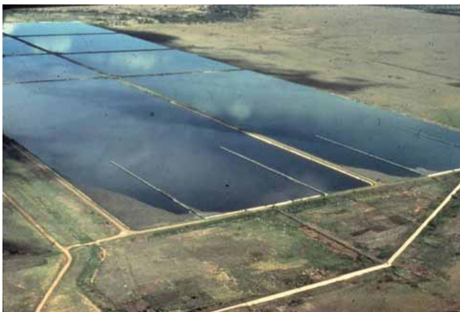
Figure 4. Phase I of the WSP system at Dandora serving Nairobi, Kenya (design flow 30,000 m 3 /d) comprising two series with a facultative and three maturation ponds. [Phase II comprises a further six series to the right of the Phase I series (design flow 80,000 m 3 /d), and Phase III will add an anaerobic pond as the first stage in the eight series (design flow about 160,000 m 3 /d).]
