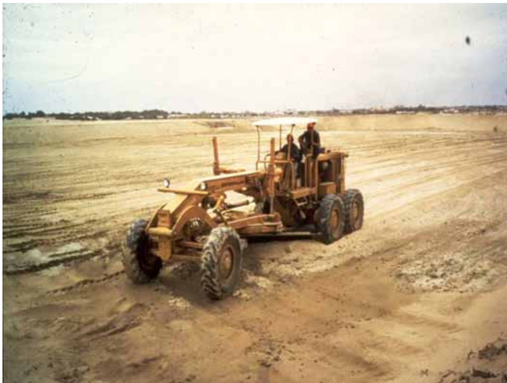
Figure 5. WSP construction – earthmoving is the main activity.
