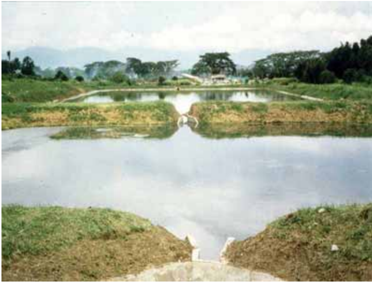
Figure 15. An example of poor inlet and outlet arrangements in a facultative ponds and a maturation ponds. They are all located directly opposite each other in the centre of the pond width (rather than in diagonally opposite corners), so maximizing hydraulic short-circuiting.
