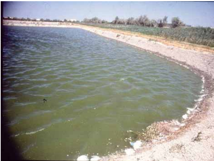
Figure 7. Embankment protection with stone rip-rap.
