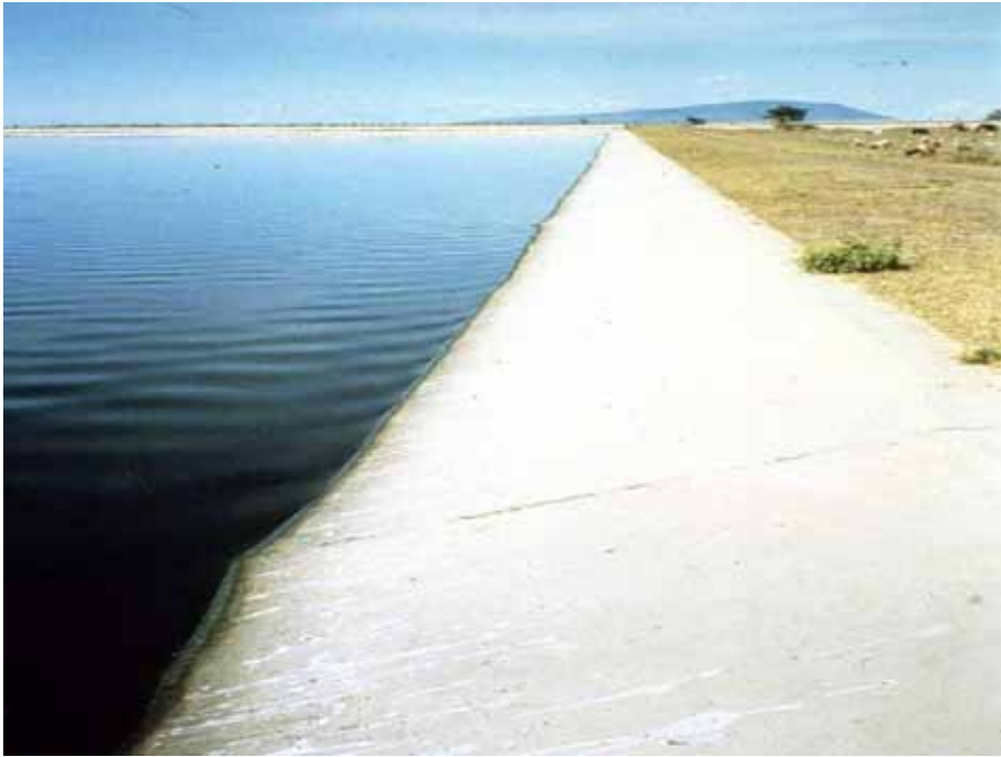
Figure 6. Embankment protection with in situ concrete slabs.
