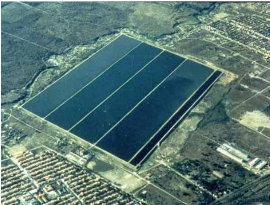
Figure 3. WSP system at Fortaleza in northeast Brazil comprising an anaerobic, a facultative and three maturation ponds (Influent flow 10,000 m 3 /day). Around half the flow is from local textile factories.
