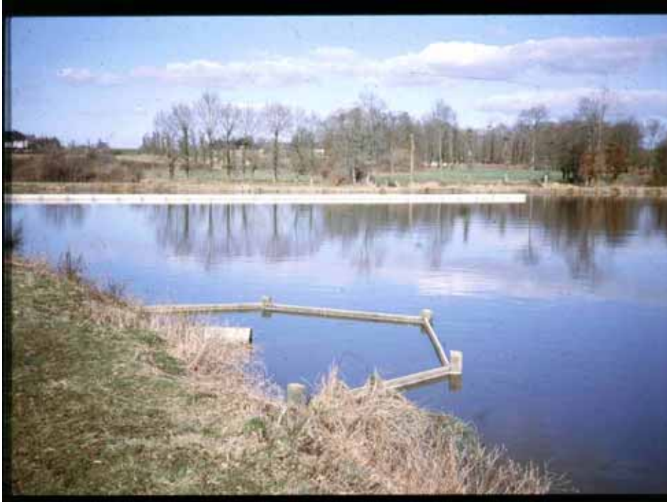
Figure 8. Pond inlet with scum box.
