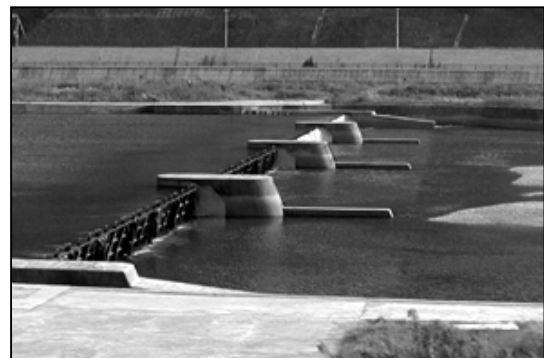
Photo 9. A modern weir in the Chikusa River (Johbaru River, Saga Pref.)
