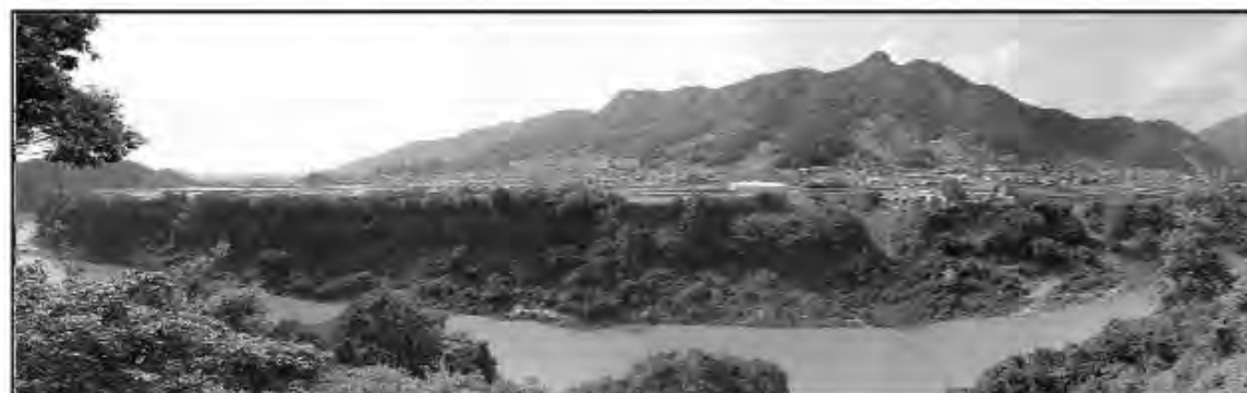
Figure 15 Landscape of dam site. According to the landscape, we decided to use straight line and low raised arch for design motif. This is the form-standard to decide the shapes of structures.
