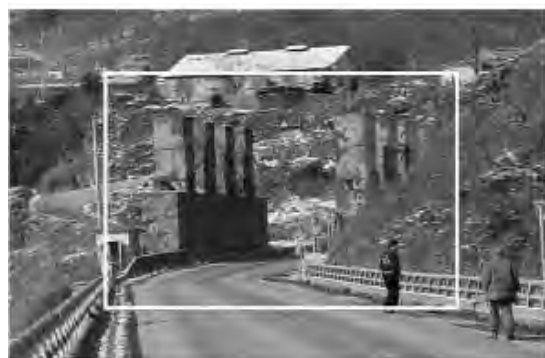
Figure 12 Military traps against the attack of tanks. In the case of emergency, supports are blown up, and heavy weights down, and close the road.
