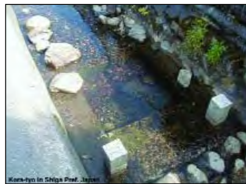
Fig. 16 : Image of [Scooping Pit] in open channel for citizens' usage (first fire-fighting phase)
