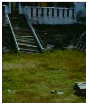
Fig. 20. Stone steps to reach the water level, here a dry urban tank, with the well in the bed exposed
