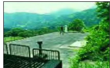
Fig. 18. 600-ton water tank
