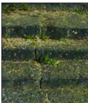
Fig. 12. Dry masonry stone steps for embankments
