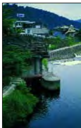
Fig. 29. Sluice gate at the Yoshida River
