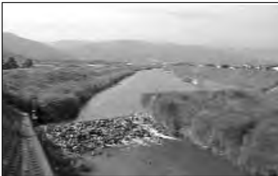
Photo 8. A traditional rubble mound weir
