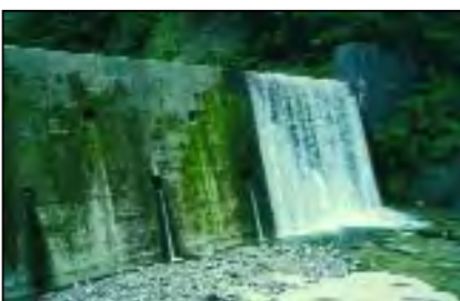
Fig. 19. Dam in the Ushikubi River
