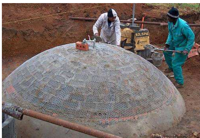
Figure 5: Construction of a fixed dome biogas plant, Lesotho (source: M. Lebofa, 2006).
