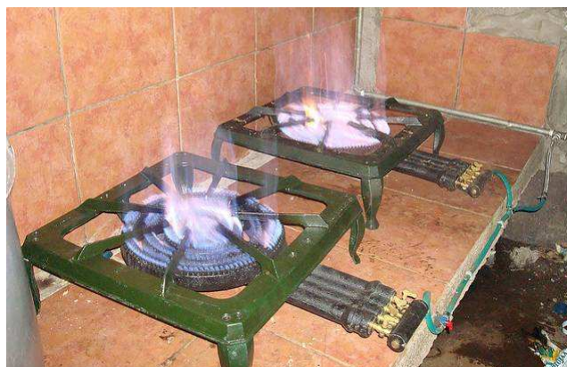
Figure 2: Biogas stove at Cachoire Girls High school, Kiambu, Kagwe District, Kenya (source: S. Blume, 2009). More photos about this project: www.flickr.com/photos/qtzecosan/collections/72157616752316076
