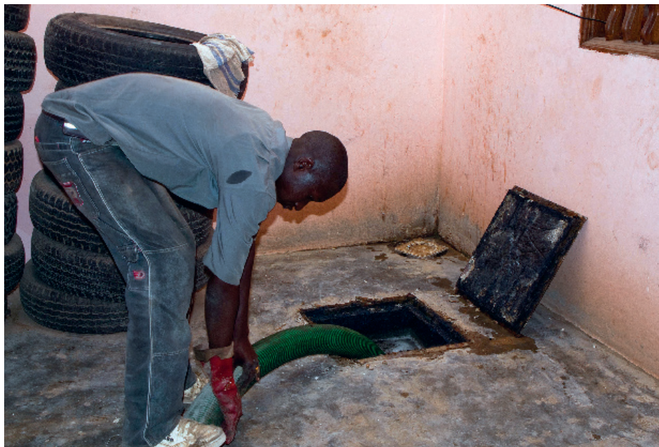
Figure 4.2 An example of an emptying operation in Dakar, Senegal where the system is located in an internal courtyard and gaining access requires cooperation with the residents (photo: Linda Strande).
