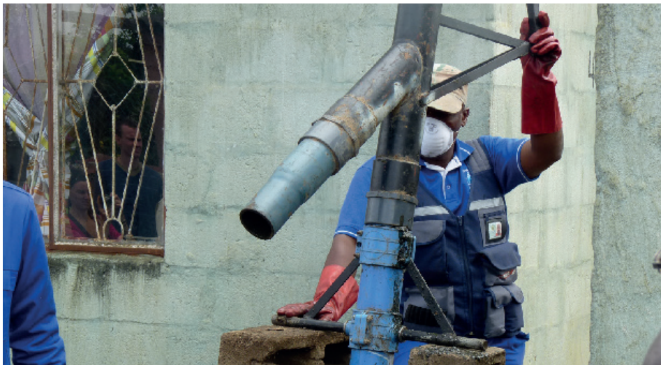
Figure 4.8 Mechanised pit screw auger in South Africa (photo: David M. Robbins).
