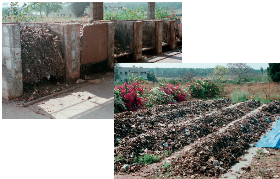
Figure 3.11 Pilot scale co-composting facility with faecal sludge and municipal waste in Bangalore, India (photo: Chris Zurbrügg).
