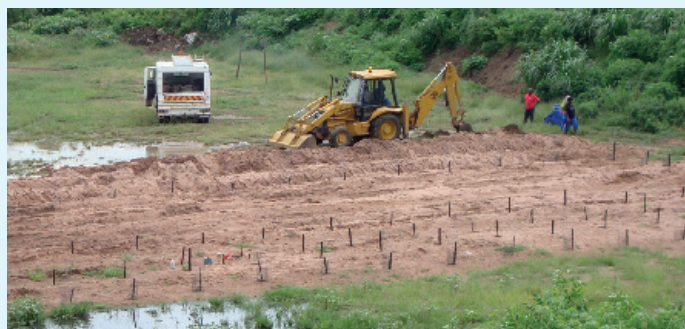
Figure 5.4 The Umlazi Deep Row Entrenchment Test Site – top the burial of faecal sludge from pit latrines in 1m deep trenches; below an overview picture of the filled trenches with trees planted on top. Groundwater wells were mapped to follow the fate of nutrients, organics and pathogens (photos: Jay Bhagwan, Water Research Council, South Africa).
