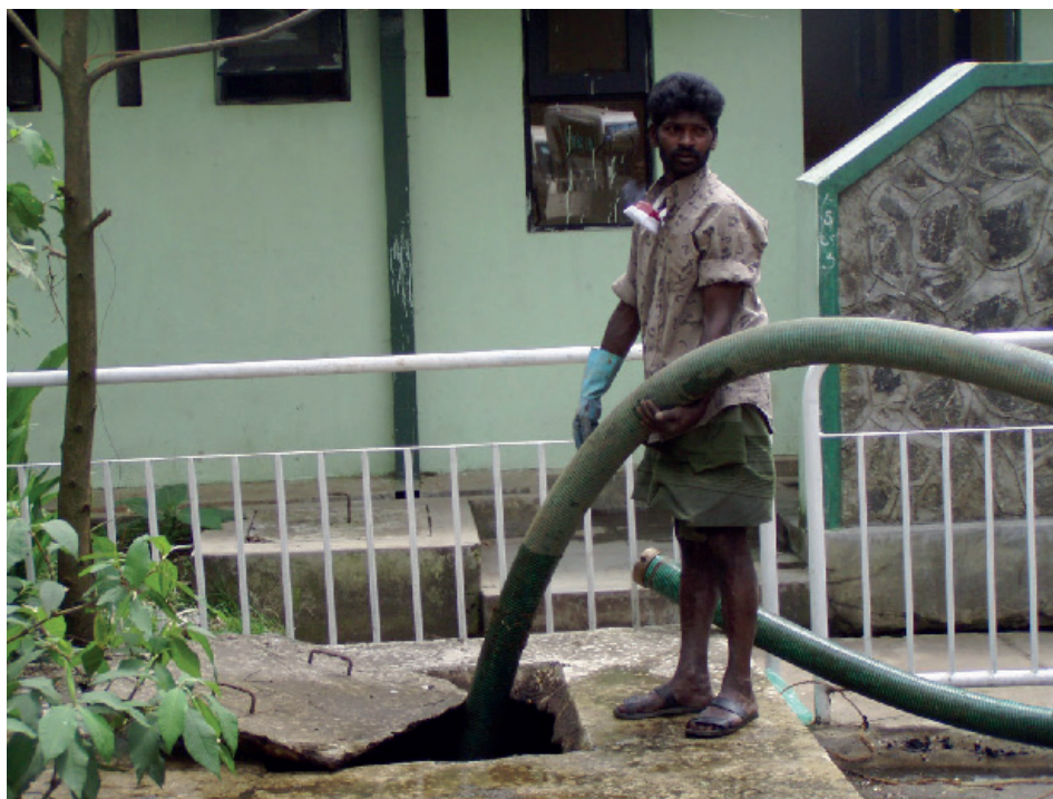
Figure 4.1 Emptying operation of faecal sludge from a septic tank using vacuum equipment. Job safety would be improved by better protective equipment (photo: David M. Robbins).
