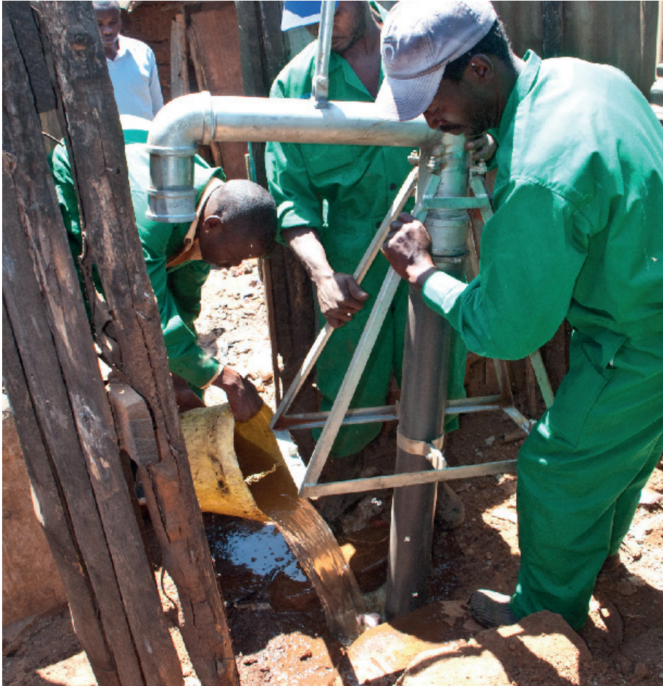
Figure 2.2 Addition of water to aid in collection of fecal sludge from a pit latrine utilising a “Gulper” in the Kibera informal settlement, Nairobi, Kenya (photo: Linda Strande).
