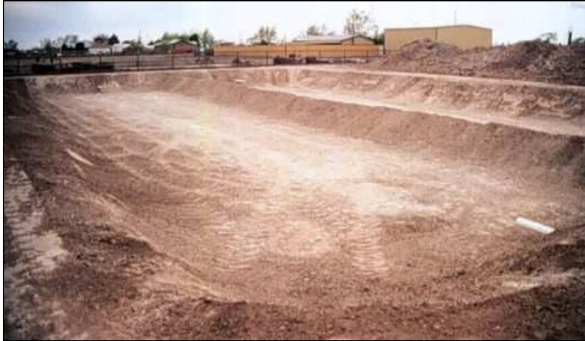
Figure 7. Excavated and graded site showing a slight slope (~1%) in the lengthwise direction of flow (Purdue 2007)
