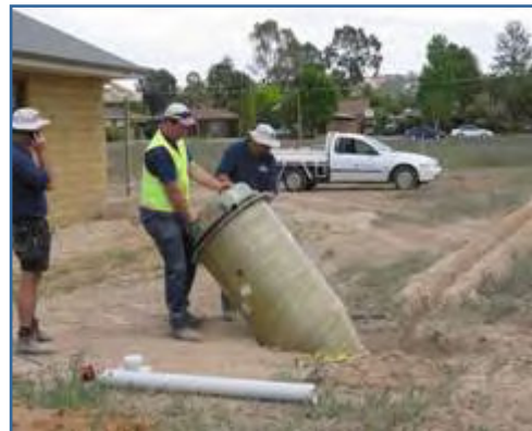
A pressure sewer unit being installed (older type)
