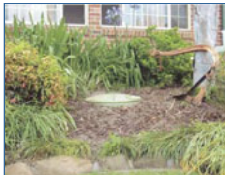
Pressure Sewer Unit Installed
