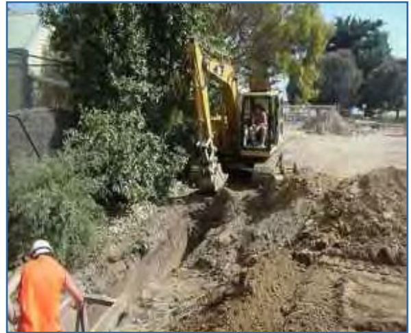
Installing a conventional gravity main.
