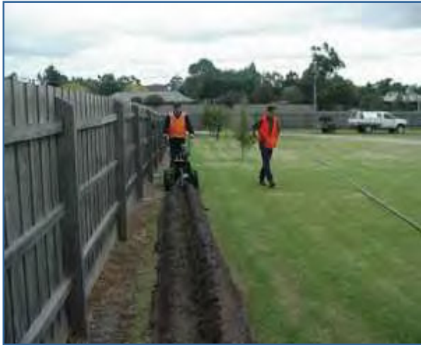
Installing a low pressure grinder pump rising main in private property.
