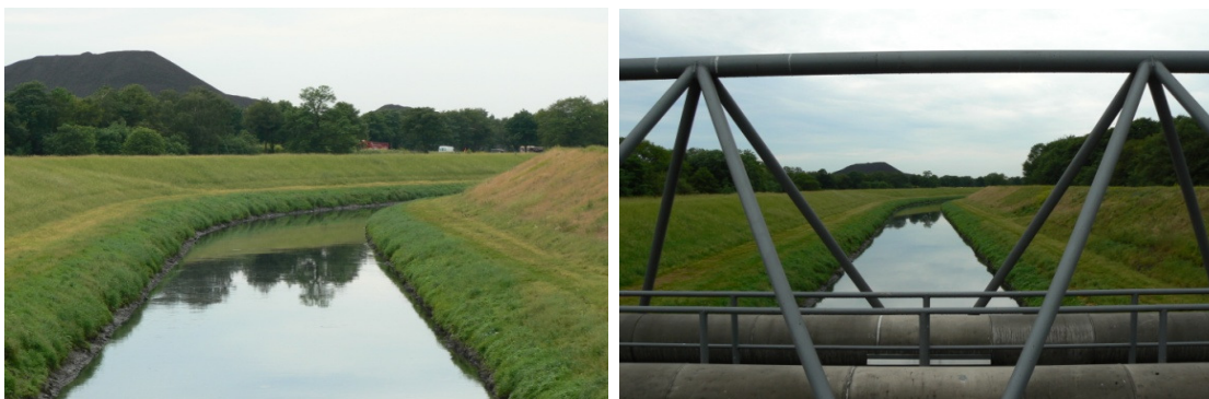
Figure 3: The straightened and channelized river Emscher carrying the sewage
