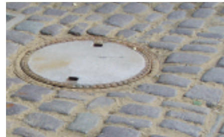
Above both: Covers are available for pedestrian (centre: G-type collection chamber) or heavy duty loading (right: Z-type collection chamber).
