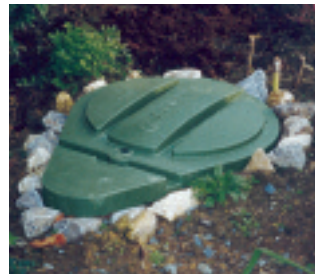
Left and centre: G- and Z-type collection chamber – The vacuum valves are installed in the valve chamber of the Roevac® collection chamber, hygienically separated from the wastewater in the sump.
