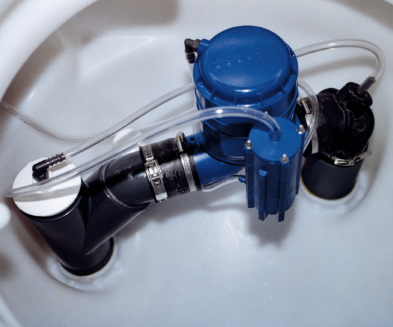
Above: 65mm dia RoeVac® vacuum valve (diaphragm type) including pneumatically
