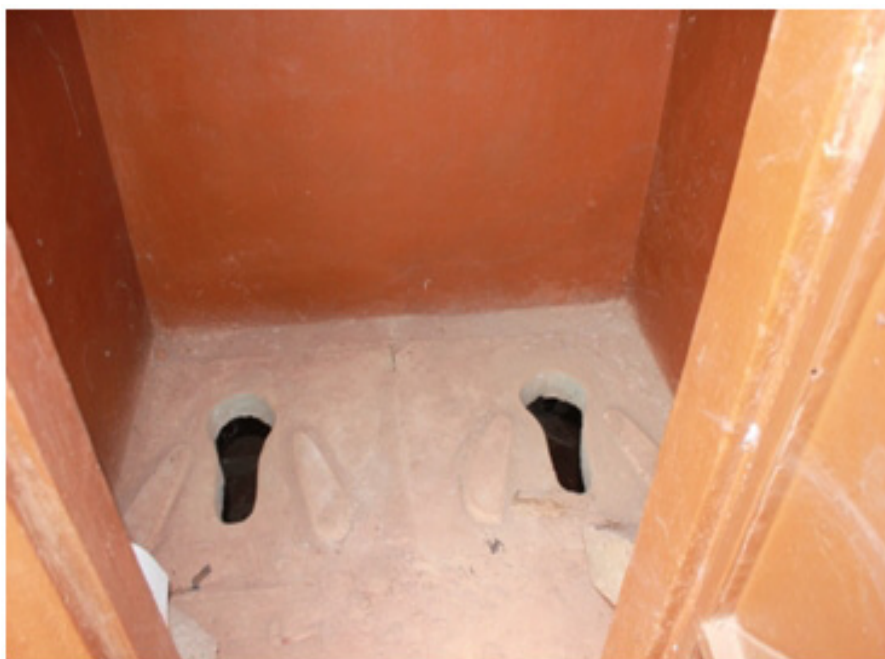
Improved school sanitation facilities maintained in a hygienic state (T. Quayle)
