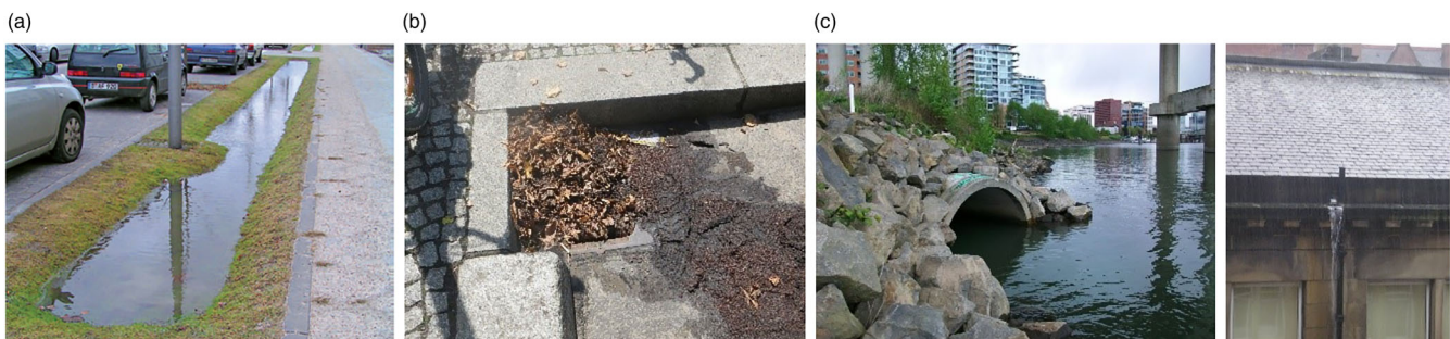
FIGURE 6 Buffers, barriers, and boosters of urban diffuse pollution: (a) swale directly after rain event, (b) blocked gully, and (c) rain gutter and storm-water outlet
