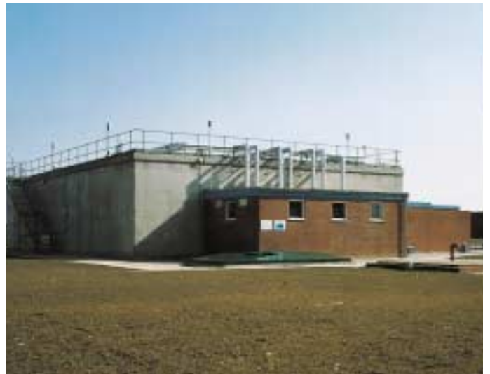
Figure 3: Contact tank with radial diffusers
