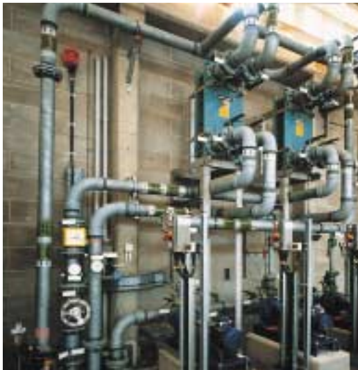
Figure 4: Cooling water system
