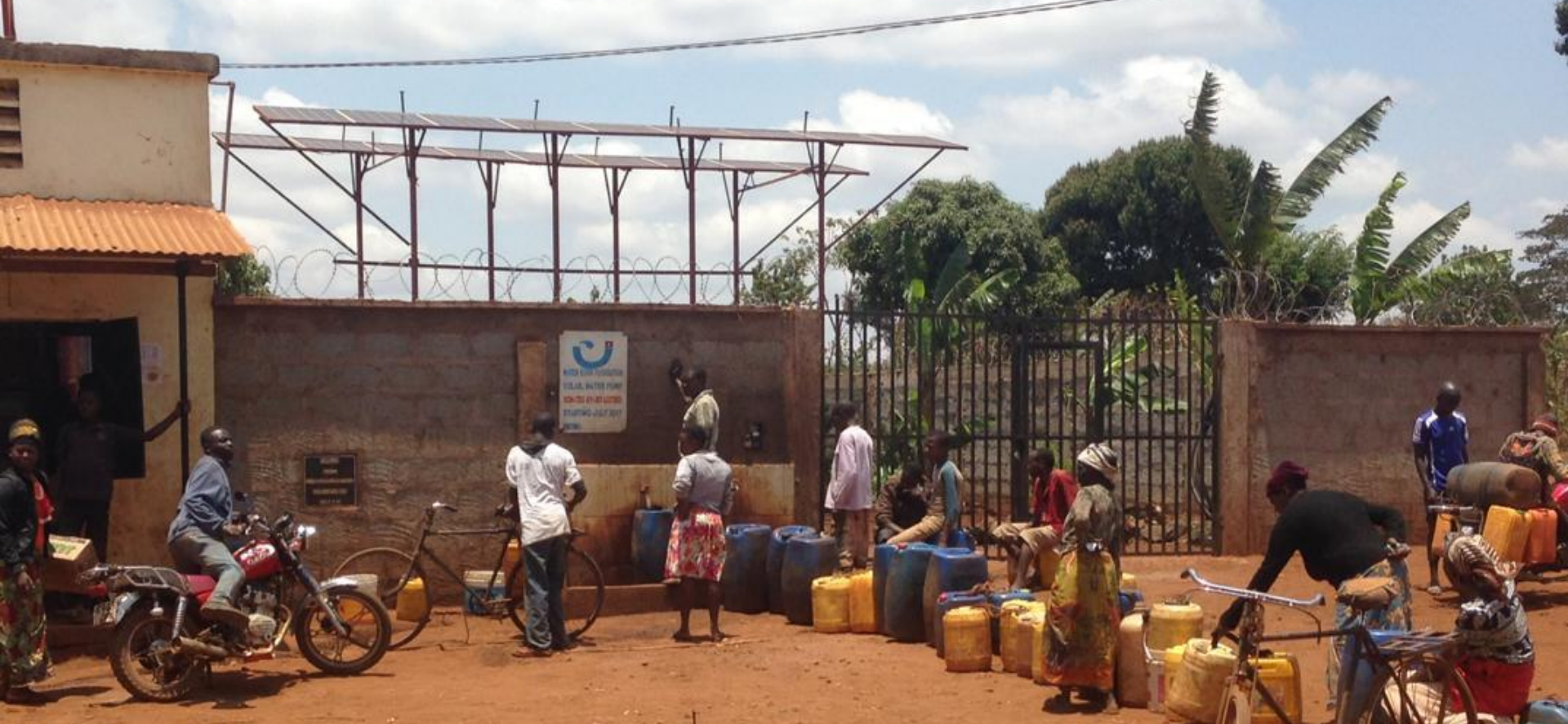
Main tapping station in Rombo
