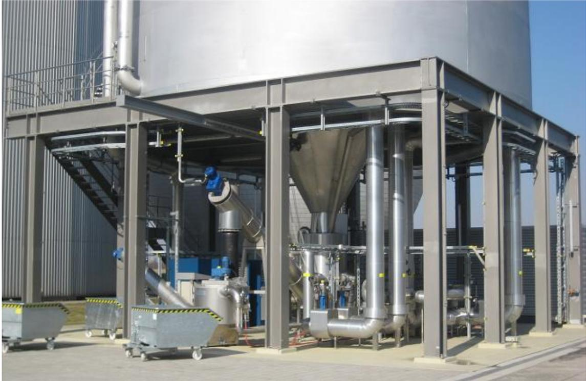
**Figure 30: The bottom of the AirPrex Reactor.**
