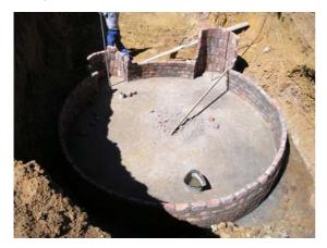
**Picture 3:** The first rows of the digester are built. The circular form is made with a lath that is attached in the middle of the foundation (radius, 25.11.2008).
