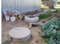
**Picture 2:** Gas outlet and dome outlet in the back (Nov. 2008)
