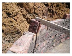
**Picture 4:** The wooden lath got a rectangular cut in order to easily keep the bricks in the right position (25.11.2008).
