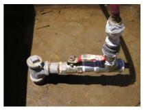
**Picture 12:** Open gas valve with connection to gas meter (9.1.2009)
