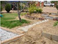
**Picture 2:** Chambers of digester, ABR and PGF (left) (Nov. 2008).
