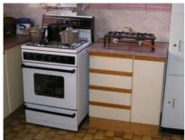
**Picture 10:** Biogas stove in the kitchen on the right side (13.1.2009)
