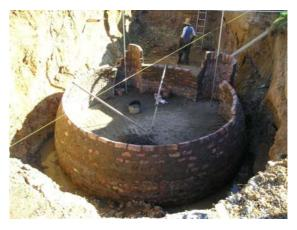
**Picture 6:** When the wall reaches a certain height respectively a certain slope hooks are required to hold the bricks in position (25.11.2008).
