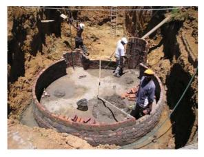
**Picture 5:** The positions of inlet and outlet chamber depend on the existing sewage pipe and the available space for ABR and PGF (25.11.2008).
