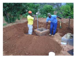
**Picture 5:** The next step consists of testing the surface of the gas storage chamber. Therefore part of the digester has to be dug free.
