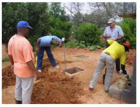
**Picture 4:** Here the gas pressure was build up manually by blowing air into the digester. This could also be done with exhaust gas of the car. Filling the inlet with water also increases the gas pressure to a certain extent (the higher the pressure the easier the detection is).
