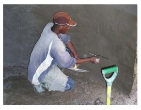
**Picture 12:** The digester is smoothly plastered from inside from the top to the bottom. Afterward the curing process starts (12.12.2008)
