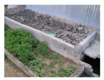
**Picture 4:** Drying bed, effluent is put on top to be dried (Nov. 2008)
