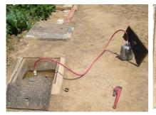
**Picture 7:** During gas flaming the iron plate protects the pipe (18.12.2008).
