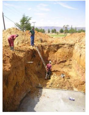
**Picture 2:** The foundation for the digester is already casted while the one for the ABR is still in preparation. Final digging and soil removal has to be done manually (21.11.2008).
