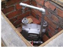
**Picture 5:** Gas meter is fixed installed (19.11.2008).
