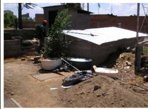
**Picture 11:** Dome inlet and outlet (lower left corner) in the front. In the background the open stable for the pigs. Pig waste water is directly flowing into dome inlet chamber. Two bowls of feedstock paper are standing next to the inlet chamber.
