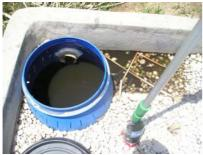
**Picture 10:** PGF outlet, effluent tank - effluent is used for irrigation (10.12.2008)
