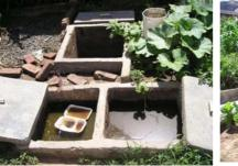
**Picture 10:** Oulet chambers of PGF, effleunt used for irrigation (13.1.2009).
