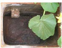
**Picture 9:** Dome outlet with scum layer (Nov. 2008).
