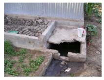
**Picture 10:** Oulet of expansion chamber, effluent enters the water canal (Nov. 2008)
