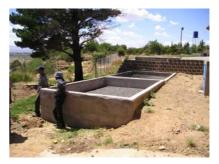
**Picture 3:** PGF in series; different size of crashed stones (Nov. 2008).
