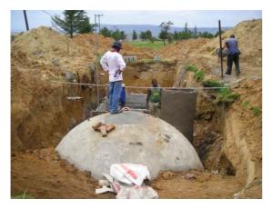
**Picture 11:** The digester is closed by installing a gas plug valve where the gas can be released. The inlet chamber is going to be finalized (10.12.2008).
