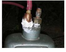
**Picture 6:** The pipe is gas tightly connected. Sealing wax is attached (8.12.2008).
