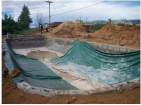
**Picture 16:** In order to protect the plaster from sunlight it gets covered. To much sunlight causes a fast drying of the plaster resulting in generating breaks (leakages, 13.1.2009).
