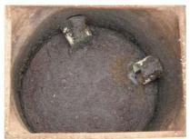
Picture 8: Dome inlet with scum layer (Nov. 2008)
