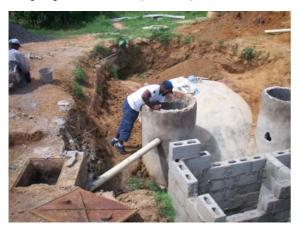
**Picture 15:** Inlet chamber gets connected with waste water pipe from school (12.1.2009).
