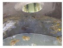
**Picture 7:** Dome inlet, water level goes down when releasing biogas (9.1.2009)
