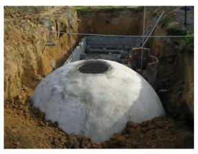
**Picture 9:** Before closing the upper part of the digester it gets smoothly plastered and partly covered with soil (8.12.2008).
