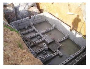
**Picture 10:** The chambers of the ABR are visible. The walls are reinforced with steel rods that are put into the brick holes and then filled with plaster (8.12.2008).
