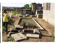
**Picture 3:** PGF with outlet chambers (Nov. 2008).
