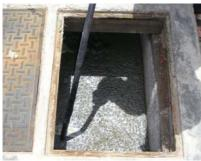
Picture 7: First chamber of ABR (Nov. 2008).
