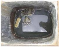
**Picture 8:** Dome outlet, some sanitary towels passed the digester (9.1.2009).
