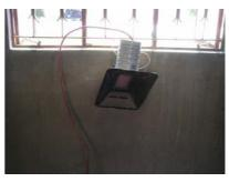
**Picture 6:** Gas heater operated with biogas (Nov. 2008).
