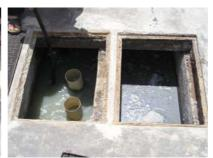
**Picture 8:** Two chambers of ABR. Two pipes that lead to water to the bottom of the chamber (Nov. 2008).
