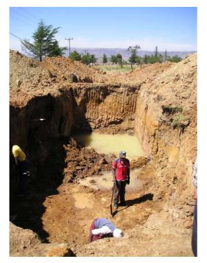
**Picture 1:** After locating the site the soil is dug out according to the project plans. In the foreground the hole for the digester and the ABR is visible, in the background for the PGF (17.11.2008).
