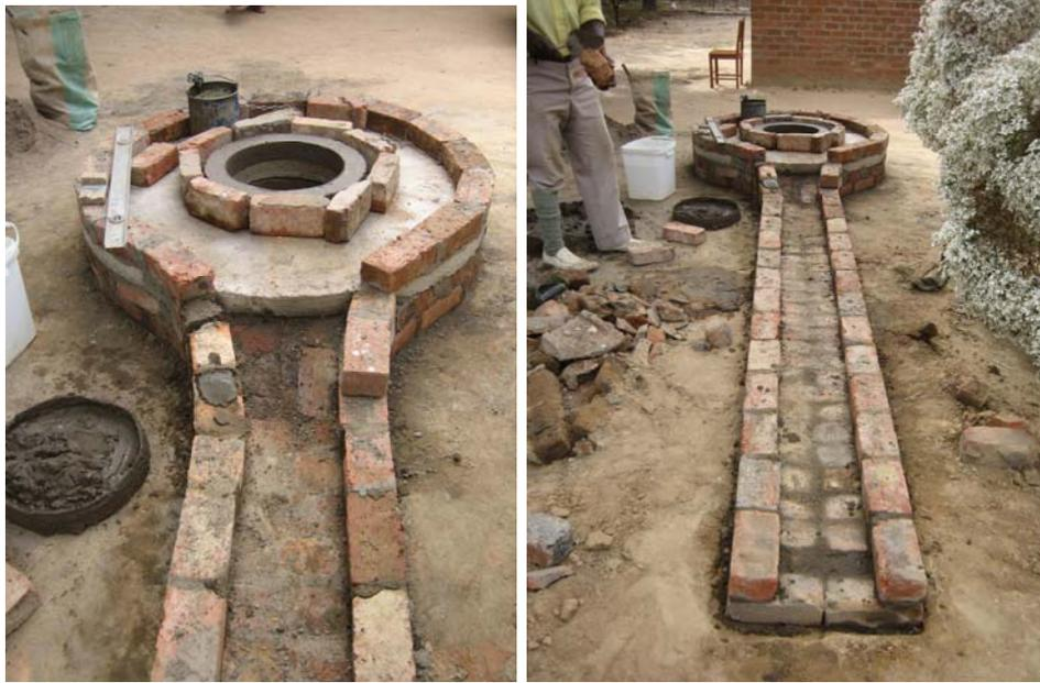
**The water run-off channel is built in bricks as shown. It is about 3m long and slopes from the well head down to a seepage area.**
