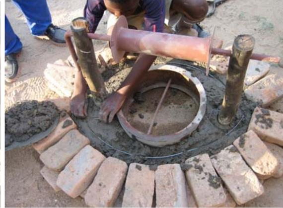
The concrete is added to the mould with plenty of reinforcing wire
