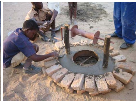
The mould is filled up so the concrete is at least 15cm deep
