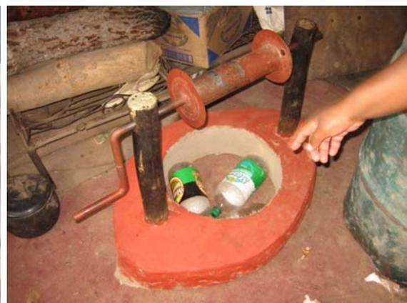
The concrete is allowed to harden a little. Then central round mould is removed followed by the windlass. The concrete work can be shaped up to be neat. The concrete anchor, supporting the two windlass support poles is left to cure for at least 2 weeks and is kept wet at all times. In the future this concrete anchor will be put to the test as the windlass is used.
