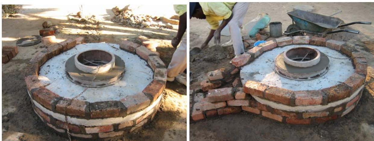
**Bricks being laid so that drained water will flow into the water channel.**
