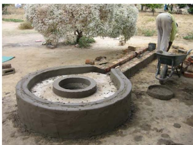
**The well head and run-off are plastered with strong cement mortar**
