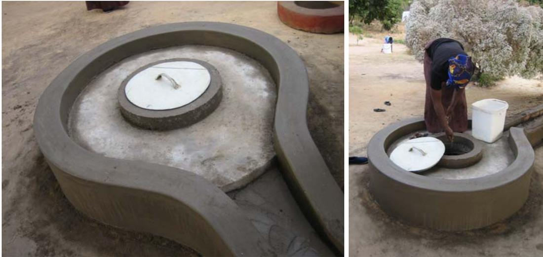
**Water can be withdrawn using the simple rope or chain and bucket from the well chamber.**
