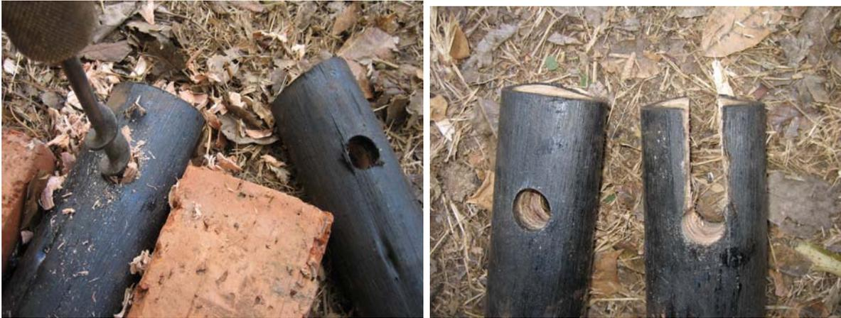
Two holes are drilled with a brace and bit 25mm wide and 75mm down through the two poles. In one of the poles the hole is opened up with a saw and wood chisel as shown.
