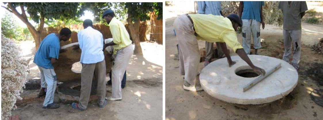
**The new well slab is placed over the original well slab in a bed of cement mortar. The slab level is adjusted so it slopes very slightly towards the side where the run-off will be built.**
