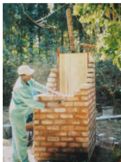
The steel frame is mounted again on the slab and the same bricks are used to rebuild the structure.
