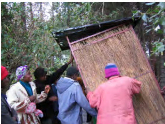
First, the structure and slab are removed from the pit which has been in use for one year. The pit contents are then covered with a good layer of soil and leaves (right).
