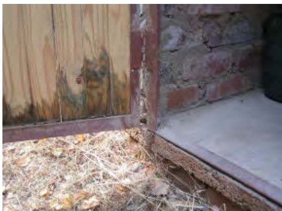
Closer views are parts of the frame. In this case the frame is made from 40mm X 40mm X 5mm angle iron. In this case the hinges are steel, but a more durable hinge can be made from car tyre. This is shown in the chapter on special construction techniques later in this book.
