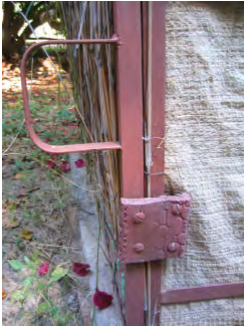
Close up of hinge and carrying handle and arrangement of steel work.
