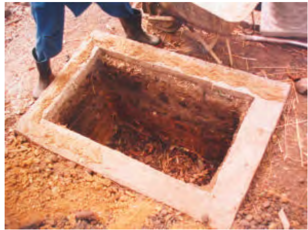
Adding dry leaves to the base of a pit helps the composting process. A full sack full or even two sacks full works well. The pit is ready – ring beam in place and leaves at bottom
