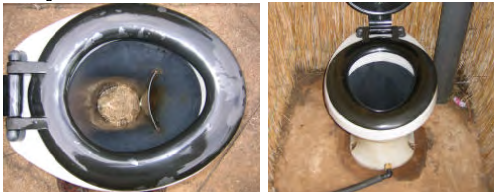
This urine diverting pedestal has been fitted to a Fossa alterna system. The urine off-take is fitted above the base of the pedestal so that the pipe can be led above the slab to the most suitable place – like a container, compost-pit or tree. The 110mm vent pipe passes through a hole made in the slab and is fitted in this case inside the toilet house.
