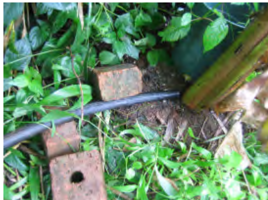
A simple structure is built around the vault for privacy and the urine pipe is led off to a banana plant close by. Structures can also be upgraded.
