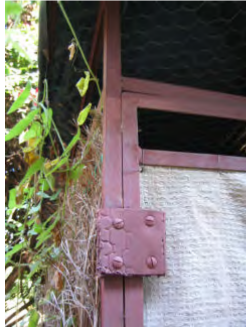
Close up of hinge and carrying handle and arrangement of steel work.
