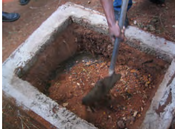
First, the structure and slab are removed from the pit which has been in use for one year. The pit contents are then covered with a good layer of soil and leaves (right).
