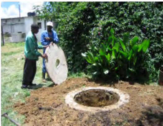
The ring beam has been embedded in levelled ground and the pit dug out to required depth. Soil extracted from the pit is placed around the ring beam. The slab is then fitted on the ring beam
