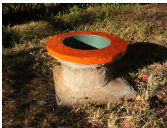
Very low cost pedestal made from a ten litre plastic bucket and cement only. It is durable and with suitable painting can be made very smart.
