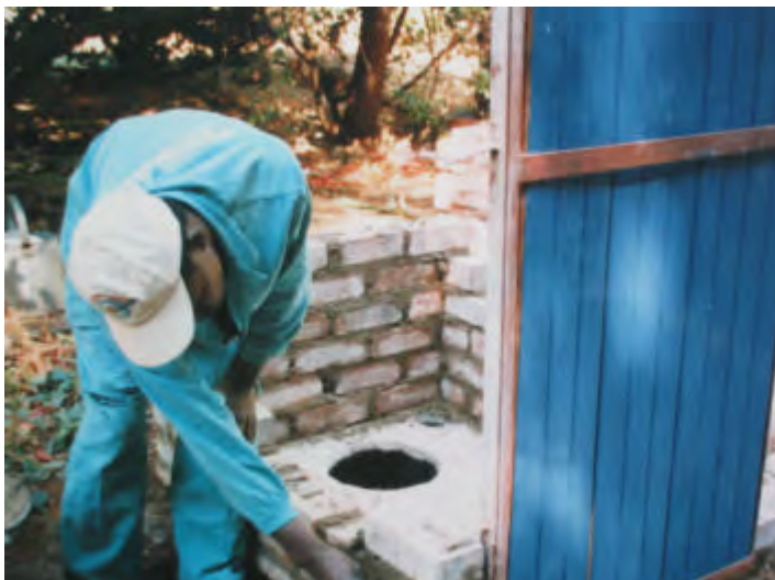
The steel frame is mounted again on the slab and the same bricks are used to rebuild the structure.
