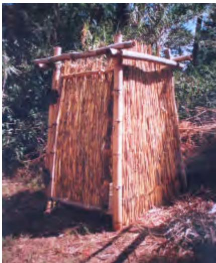
Structure made of bamboo and reeds. The four main bamboo uprights are anchored in the ground. They can be protected to a certain extent from ants with old engine oil or wood ash. The hinge for the door is made of old car tyre, as shown on the right. This material makes an effective and durable hinge.
