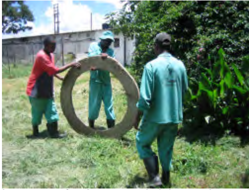
Round concrete ring beams and slabs can be made off the site and rolled into position as these photos show. In this case the larger ring beam (ID 1 metre) is being rolled onto site and fitted with a 1.15m diameter slab.
