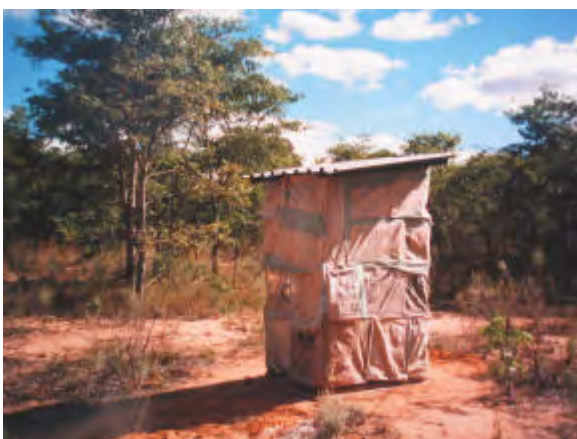
Structure using small gum poles and old cement packets – also with a door Photo taken at Kufunda Village Ruwa. Thanks to Marianne Knuth. Moving an Arborloo superstructure in Maputaland, South Africa. Note the wooden structure has legs. Thanks to Dave Still and Stephen Nash of Partners in Development.
