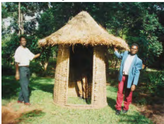
Woven basket superstructure from Malawi. Thanks to Steven Sugden and WaterAid. Woven basket structure on Arborloo in Northern Malawi. The door is made from sacking. A neat and effective unit. Photo: thanks to Jim McGill, Embangweni eco-san project.
