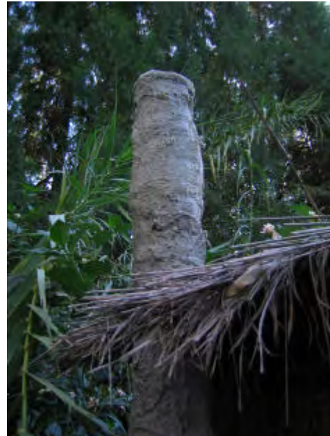
A durable home made vent pipe constructed from Hessian and a sand cement slurry with some wire reinforcing. Very effective and longlasting.
