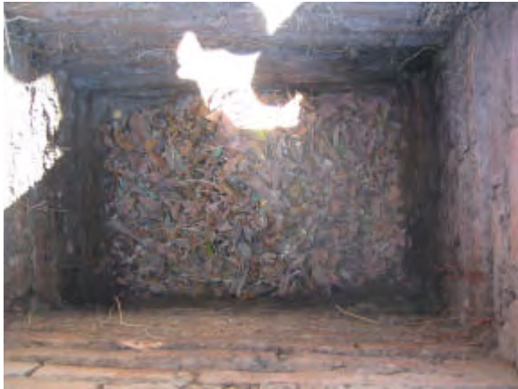
The layer of leaves at the base of the pit. Note that small roots have invaded the pit, even through the brickwork to find the nutrients available in the composting excreta. On the right, the superstructure is now moved from the now almost full pit and placed on one side. The home made pedestal can be seen.
