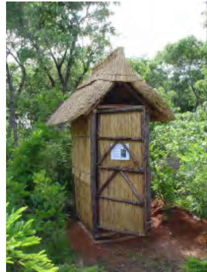
Left, the simplest superstructure – poles and grass – no door - no roof. Thanks to Jim Latham, Eco-Ed Trust. Right, more sophisticated pole and grass structure with door and roof. Durable door hinges can be made with cut sections of car tyres. Photo taken at Kufunda Village, Ruwa.
