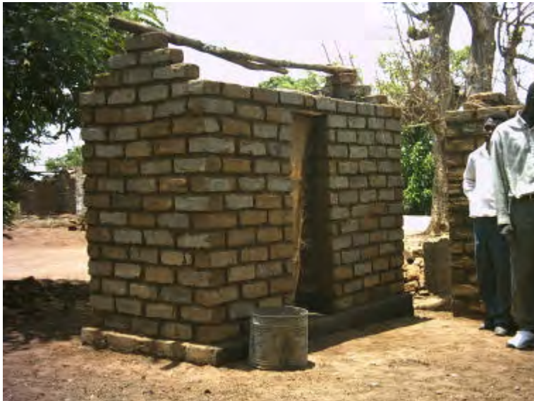
Very neat Fossa alterna constructed in peri urban settlement near Lilongwe with support from WaterAid. The roof has still to be added. On the right a view of the interior with round domed slab.
