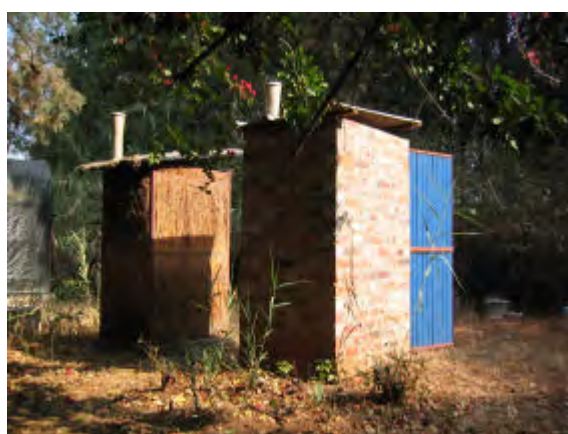
After the brickwork is complete, the roof, asbestos pipe and pedestal can be put back in place. The operation takes about 6 hours. If the pits are changed once every 3 – 5 years, this is not a huge expenditure of time and effort. Everything is recycled, even the material in the pit, which is dug out once the time has come to change sides again.
