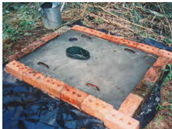
The addition of concrete is complete. Half the mix is added first, the reinforcing wire is laid, followed by the remaining concrete which is smoothed down. The handles are added by pushing them into the concrete mix. A little extra cement can be added around each handle to increase the strength of the concrete at this point. Finally the slab is smoothed down flat with a steel float and left to cure.
