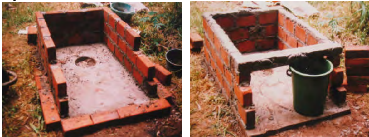
Stages in making the vault. The brickwork
