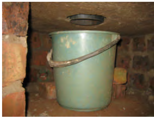
The one metre diameter slab has been fitted and bonded on top of the round vault in cement mortar and a urine diverting pedestal fitted. This could also be a squatting type urine diverting platform. The bucket is located in position under the urine diverting pedestal with some bricks.
