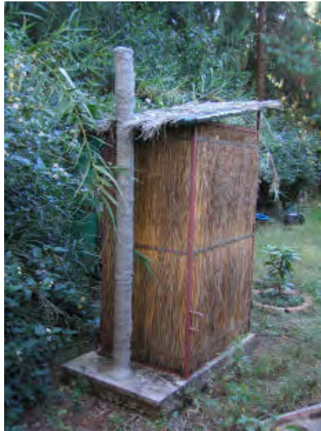
A durable home made vent pipe constructed from Hessian and a sand cement slurry with some wire reinforcing. Very effective and longlasting.
