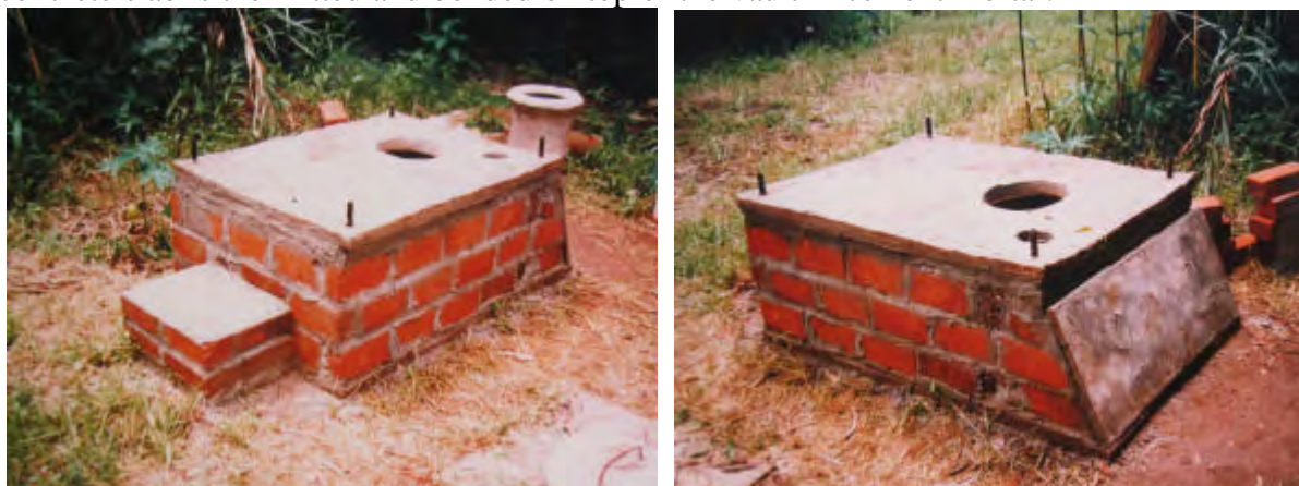
The vault access slab and the toilet slab have now been fitted. The superstructure must now be made.
