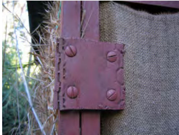
Photos of the steel frame Arborloo structure with grass walls and door made of sacking cloth. The vent pipe is a low cost home-made type made by wrapping plastic sheeting around a PVC pipe, then applying hessian and cement slurry. The structure has a door with car tyre hinge (see close up).
