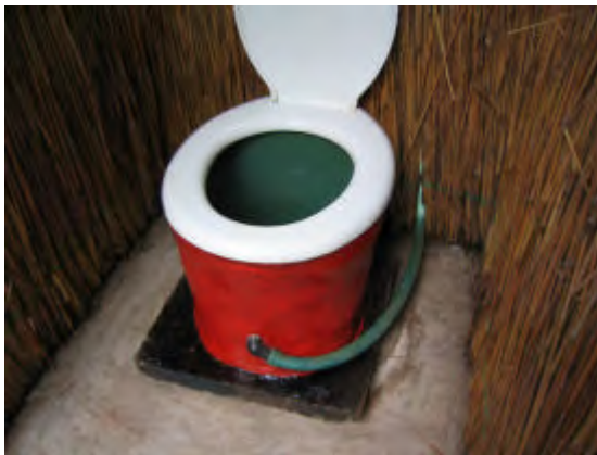
The urine diverting pedestal can be fitted into a single or double vault dehydrating or composting toilet. It can also be fitted over a shallow pit toilet. The urine pipe can be led into a soakaway or into a vegetable garden, preferably beneath ground level. It can also be led to a tree like a banana, as shown above. The urine can also be led to a plastic container placed in a hole dug in the ground. It is advisable to protect the pipe in some way by covering with soil etc. Here the pipe is exposed for the photo.
