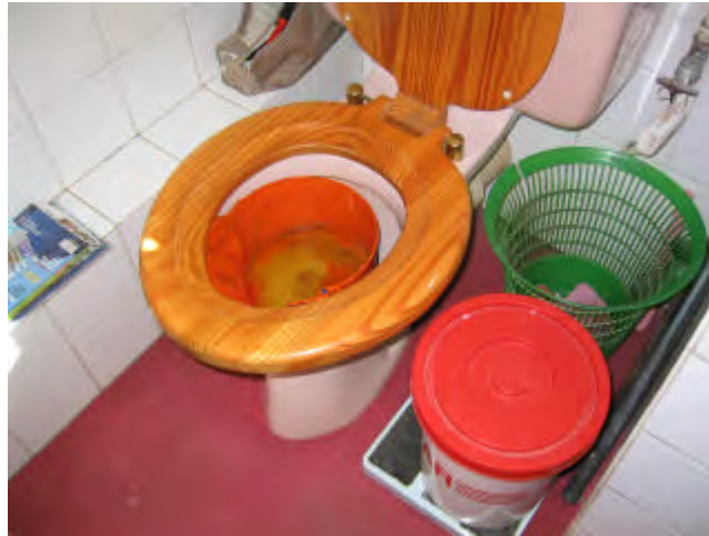
On the left a 10 litre bucket is placed beneath a pedestal which helps women to collect urine. On the right a urine collector shaped from a plastic bucket is used to collect urine from a standard flush toilet.
