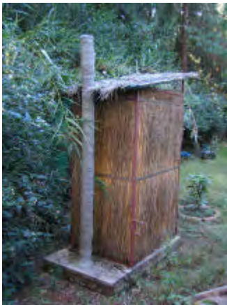
Photos of the steel frame Arborloo structure with grass walls and door made of sacking cloth. The vent pipe is a low cost home-made type made by wrapping plastic sheeting around a PVC pipe, then applying hessian and cement slurry. The structure has a door with car tyre hinge (see close up).
