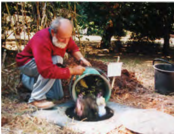
Tipping the contents of the bucket from a UD toilet into a small shallow pit for processing. The shallow pit is covered with a concrete lid with hole which is itself covered. On the left three cement jars are shown. The one actively being filled is covered with an attractive painted concrete cover.
