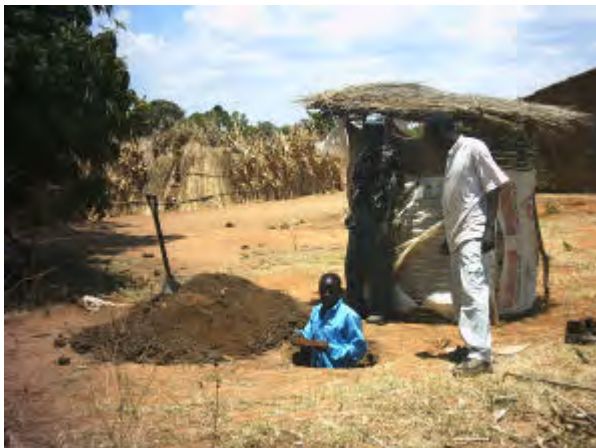
Excavation of Fossa alterna pit in Embangweni. In this case the structure is a simple bamboo portable unit which is moved from one pit the other. The ground is very firm in this locality and no ring beam or pit lining was used. The pit took less than 30 minutes to excavate and the entire operation of excavating and moving the slab and structure to the newly excavated pit took less than one hour. On the right dried leaves are being placed down the new pit. These help to compost the excreta like the soil which is added.
