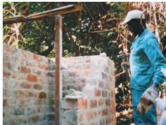
The roof is fitted after completion of the brickwork and door fitting. An asbestos pipe will also be fitted. Photo on right shows first stage of dismantling. The pipe, pedestal and roof have been removed. Now the brickwork is taken apart.
