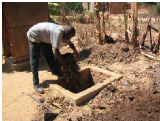
Adding leaves to Fossa alterna pits. On left at Woodhall road, on right at Epworth. Adding dried leaves to shallow pits used in the Arborloo and Fossa alterna helps the composting process considerably.
