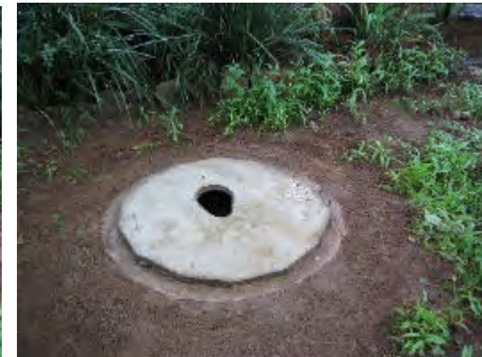
The one metre diameter slab fitted to matching ring beam.
