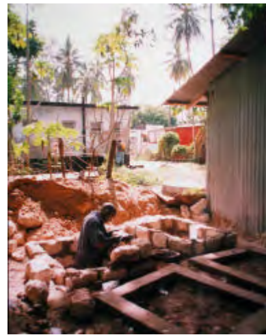
Delegates at eco-san workshop in Mombasa construct concrete ring beams within wooden frames for Fossa alterna at the Mtomondoni Primary School (left). On the right the two pits of a Fossa alterna are lined with coral limestone blocks from the base in very loose sandy soil near a beach site at Mombasa.
