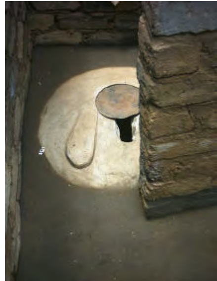
Very neat Fossa alterna constructed in peri urban settlement near Lilongwe with support from WaterAid. The roof has still to be added. On the right a view of the interior with round domed slab.
