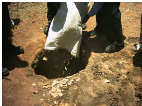
Excavation of Fossa alterna pit in Embangweni. In this case the structure is a simple bamboo portable unit which is moved from one pit the other. The ground is very firm in this locality and no ring beam or pit lining was used. The pit took less than 30 minutes to excavate and the entire operation of excavating and moving the slab and structure to the newly excavated pit took less than one hour. On the right dried leaves are being placed down the new pit. These help to compost the excreta like the soil which is added.
