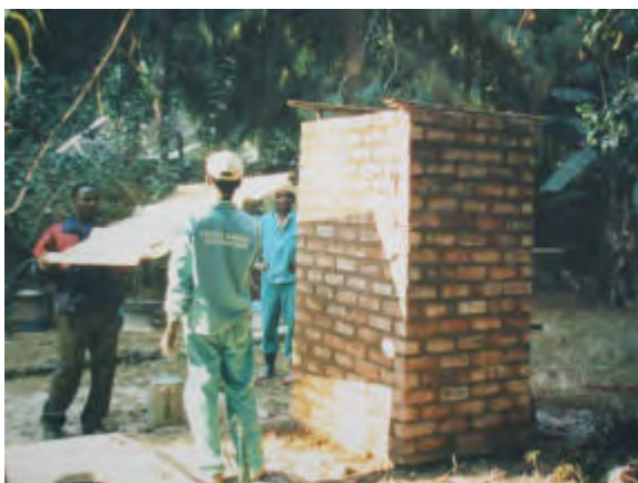
After the brickwork is complete, the roof, asbestos pipe and pedestal can be put back in place. The operation takes about 6 hours. If the pits are changed once every 3 – 5 years, this is not a huge expenditure of time and effort. Everything is recycled, even the material in the pit, which is dug out once the time has come to change sides again.
