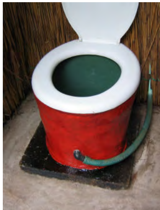
Left: Diagram showing effect of vent pipe on controlling odours and flies. Right: A urine diverting pedestal with above slab urine take-off. This type is suitable for upgrading shallow pit composting toilets like the Fossa alterna to urine diversion. Pits under urine diverting pedestals are drier and this helps to control flies and odours.
