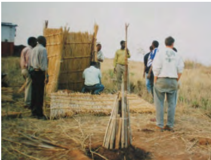
On the left - building an Arborloo near Lichinga. An Arborloo pit is just been topped up with soil and a tree planted near the foreground. On the right – the two pits of the Fossa alterna , one is partly excavated.
