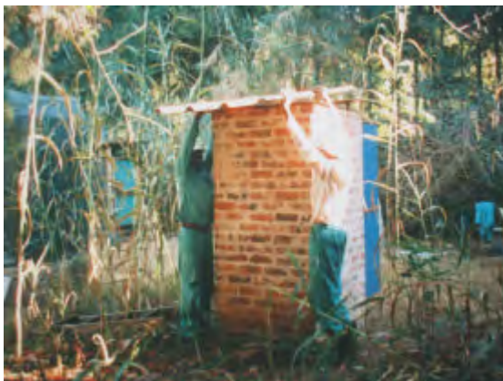
The roof is fitted after completion of the brickwork and door fitting. An asbestos pipe will also be fitted. Photo on right shows first stage of dismantling. The pipe, pedestal and roof have been removed. Now the brickwork is taken apart.
