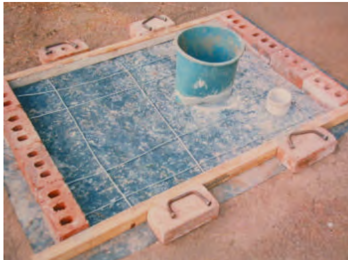
Photo of slab mould made of bricks and wooden shuttering. The eight pieces of 3mm reinforcing wire have been cut and laid on the plastic ground sheet. Four carrying handles have also been prepared. A 10 litre bucket with the base removed has been shaped by drawing in the two sides with wire. A 75mm length of 110mm pipe has also been cut to make the hole for the vent pipe. Thus all has been prepared for the addition of the concrete.
