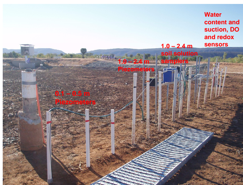
Figure 6 Observation well RN17948, shallow piezometers, suction cups, tensiometers, soil water content sensors, dissolved oxygen and Eh sensors located in RB4
