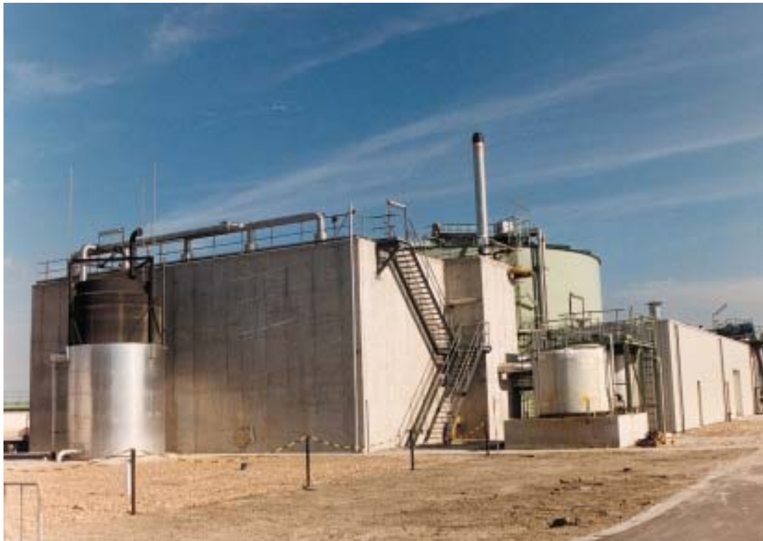
Figure 9. UASB reactor at Cerestar, Sas van Gent, The Netherlands. Photo by courtesy of Biothane Systems International.
