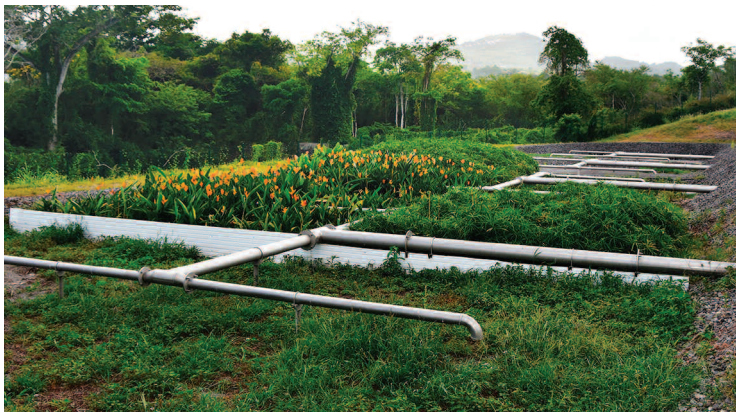
Figure 19. Partitioning—example at the Taupinière facility (Martinique). In the foreground, the filter has been partitioned using corrugated sheeting. A flange has been fitted to shut off the redundant feeding headers designed to serve the half-filter that is not yet in service. In the background, the cells that make the facility's second stream are not yet in service and have not yet been planted.
