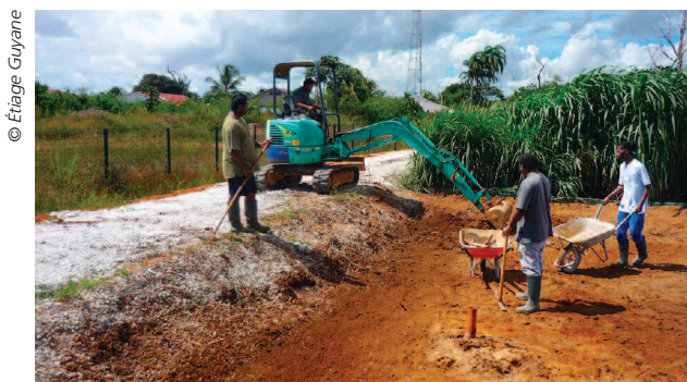
Figure 11. Desludging operation in French Guiana on Bois d'Opale 1. This sludge can be reclaimed for use in agriculture (Epnac, 2014).
