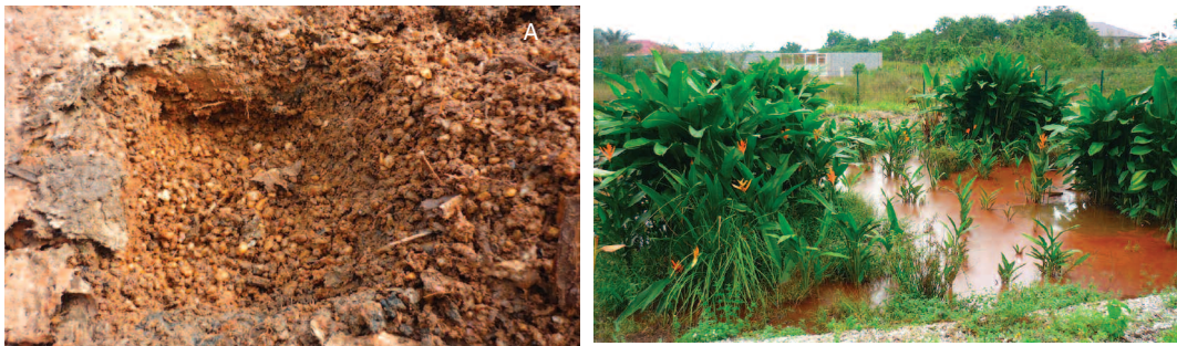
Figure 28. Bois d'Opale 1 filter clogging caused by laterite.
