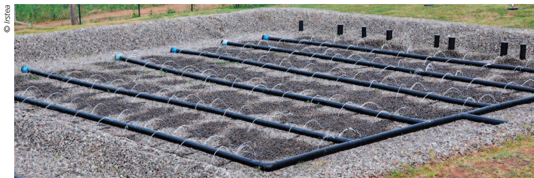
Figure 8. Feeding on second stage of the Mansarde Rancée (Martinique) facility before planting, February 2014.
