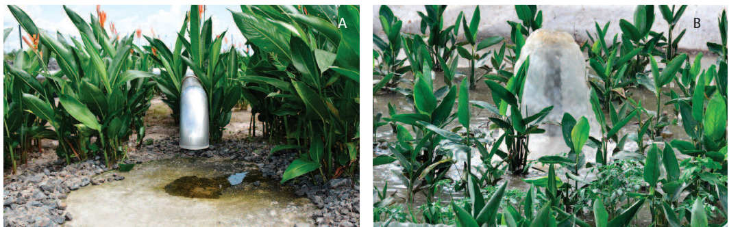
Figure 21. Elevated headers with the anti-scouring sheet (at left) or buried headers mid-feeding (at right).
