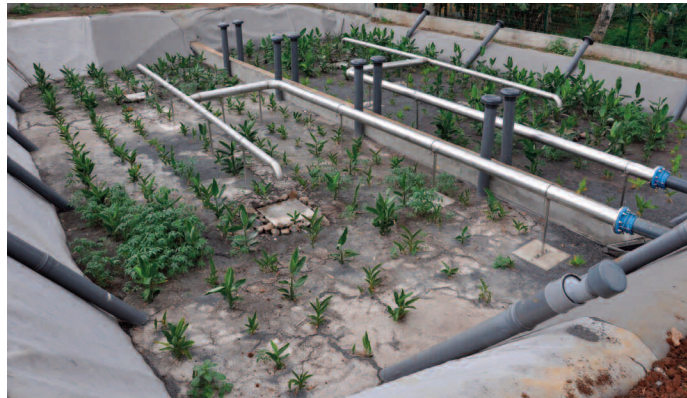
Figure 20. Partition wall separating two filters inside the same cell. Note that it could have been stacked a little higher (20–30 cm) to accommodate a higher freeboard. Champ d’Ylang 1 facility, at its inauguration in November 2015, on Combani commune (Mayotte).
