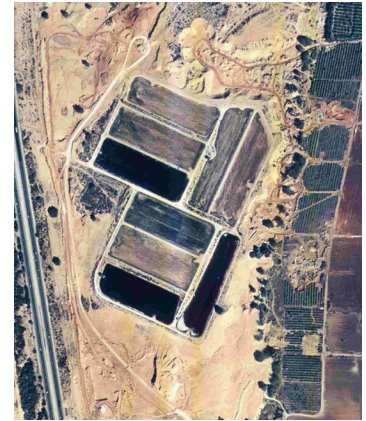
SAT soil percolation zone (Source: Mekorot)
