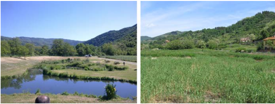
Figure 6.8 Case study 6 – Dicomano Wastewater Treatment Plant (Italy).
