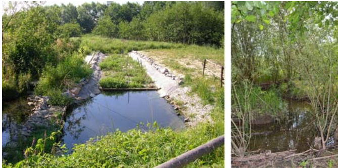
Figure 6.10 Case study 8 – Multifunctional water reservoir in Ljubljana (Slovenia).
