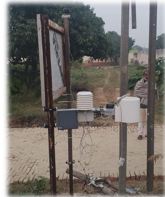
Monitoring Equipment wfSRC System
