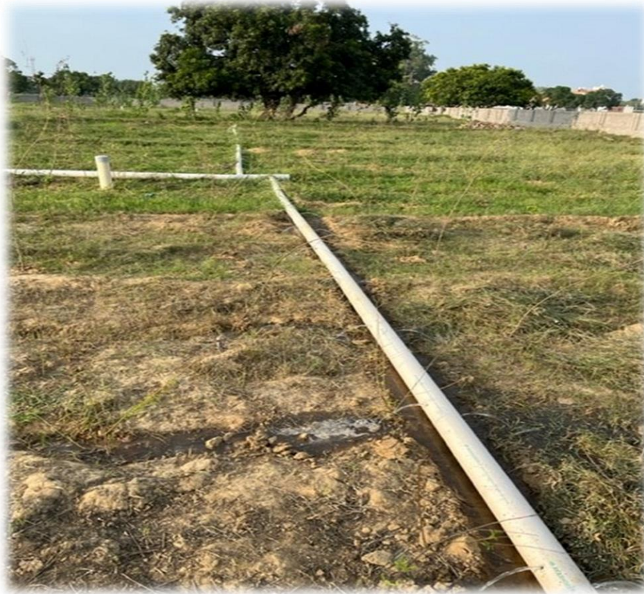
Irrigation System Installation
