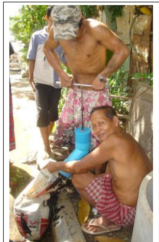
Figure 4 - First trials of the Gulper on a small drain interceptor pit in Phnom Penh by a father and son team
