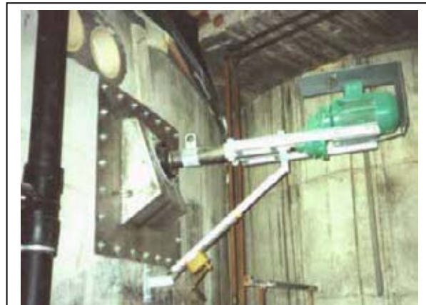
Figure 19: Stirring device for a european biodigester
