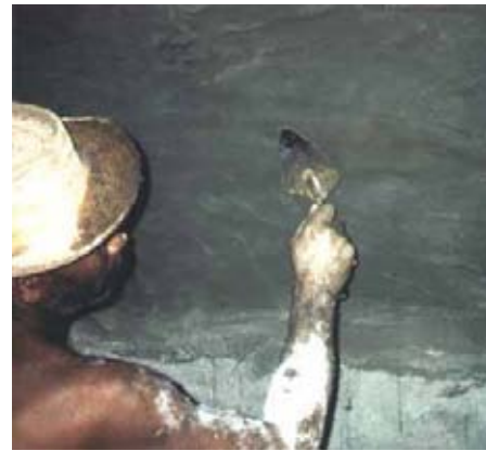
Figure 40: Inside plaster of the gastight section of a fixed dome digester
