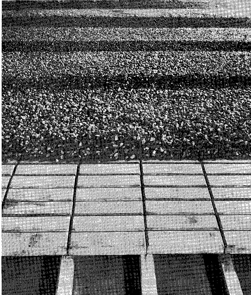
Municipal Waterworks, Amsterdam
