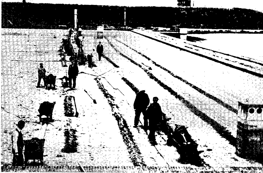
Municipal waterworks, Amsterdam
