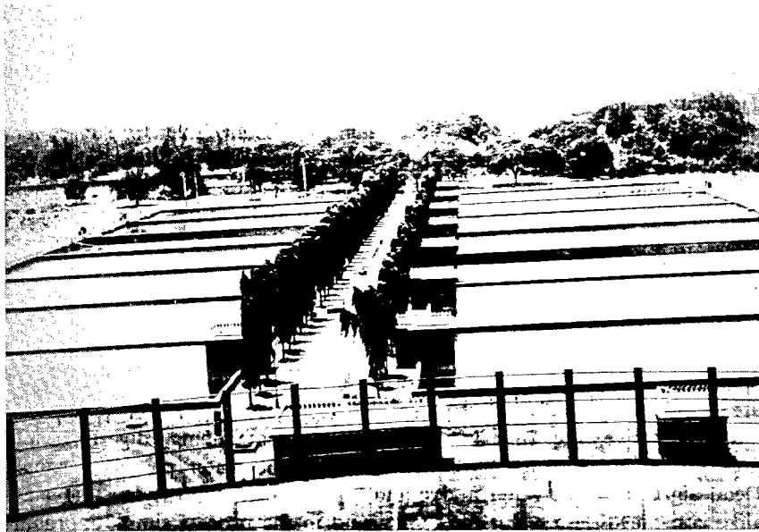
FIG. 2. SLOW SAND FILTERS AT MADRAS WATERWORKS, INDIA
