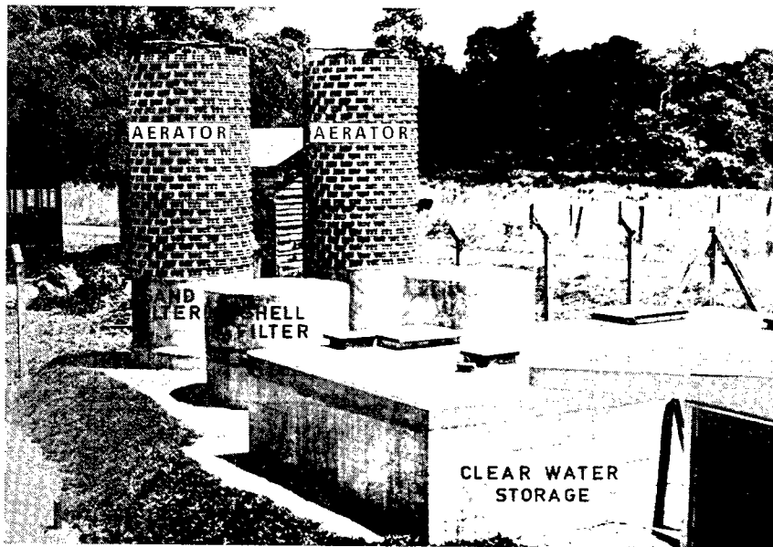
FIG. 15. PILOT PLANT IN SURINAM USING SMALL CIRCULAR FILTERS
