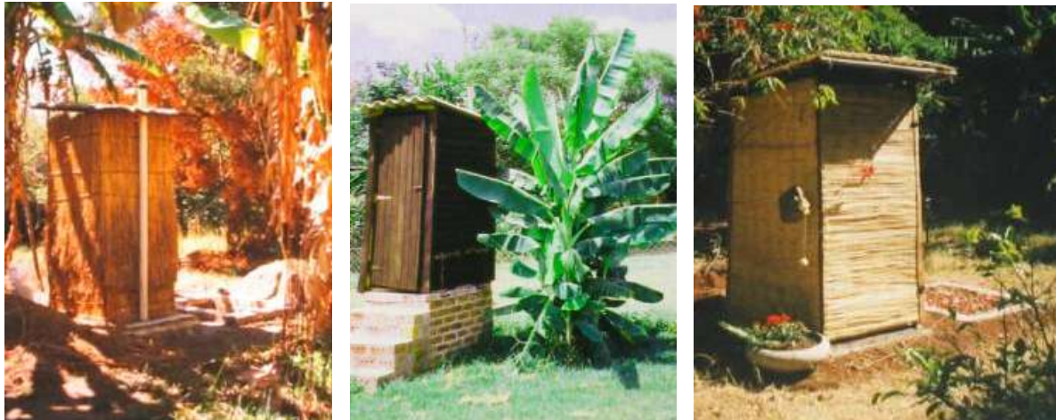
SON-MIST – movable toilet house structures, making way for fruit tree or compost production
