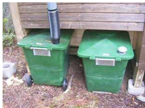
Figure 16. Movable ventilated collecting bins with overflow for leachate discharge (source : PikkuVihreä, Finland).
