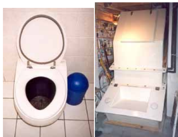
Figure 7. Left: Dry toilet with removable insert and sealed toilet seat. Right: Insulated single-vault composting container with upper lid for maintenance and lower lid for discharge and working platform (both Hamburg-Allermöhe, Germany, source: Berger and Lorenz-Ladener, 2008).
