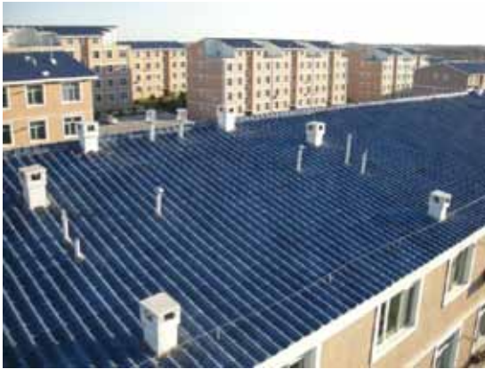
Figure 17. Part view of the multi-story houses in Dong Sheng, showing vent pipes on the roof from the ventilation system (photo : W. Berger, 2009).
