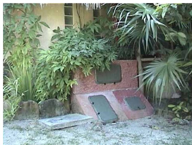
Figure 9. Owner-built single-vault composting toilet with built-in toilet connection and outside access for maintenance and discharge (Puerto Morelos, Mexico) (source: The ReSource Institute, http://www.riles.org/projmex.htm ).
