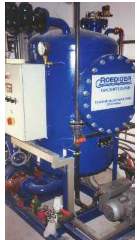
Figure 7: Prefabricated compact vacuum station (Mosel)
