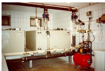
Bio-reactor for 6 apartments
