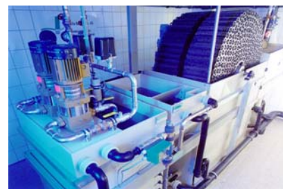
Rotating biological contactor for 24 apartments
