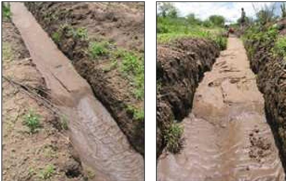
**Figure 2-9:** *Deposition of coarse sediments behind an obstruction in a small manmade drainage channel*
