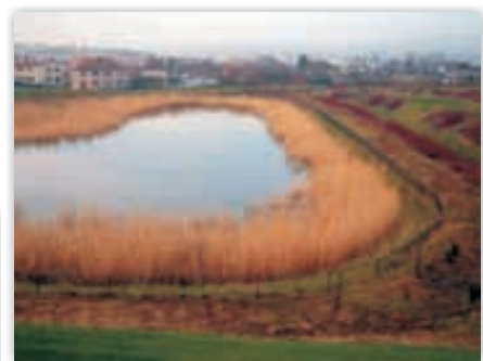
Retention Pond, Scotland
