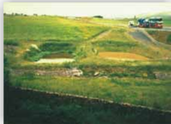
Retention Ponds, Operation Stage, M74, Scotland
