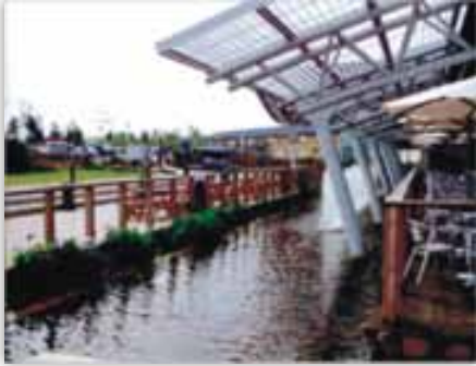
M42 Motorway Services
