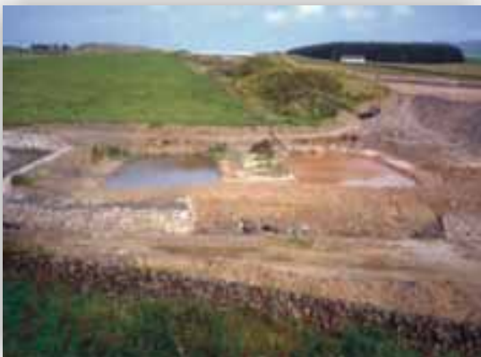
Retention Ponds, Construction Stage, M74, Scotland
