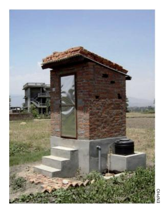
**An EcoSan toilet in Siddhipur** – The dehydration vaults are made of concrete, the superstructure of brick masonry. The urine is diverted into a 100 L PP tank adjacent to the construction
