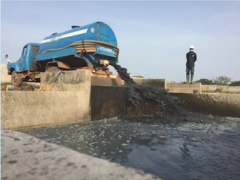
Figure 2.5.3 Discharge of faecal sludge collected and transported from households into the inspection chamber at the Korhogo faecal sludge treatment plant.
