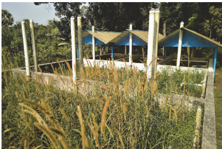
Figure 2.3.7 Faecal sludge treatment plant in Jhenaidah, Bangladesh.
