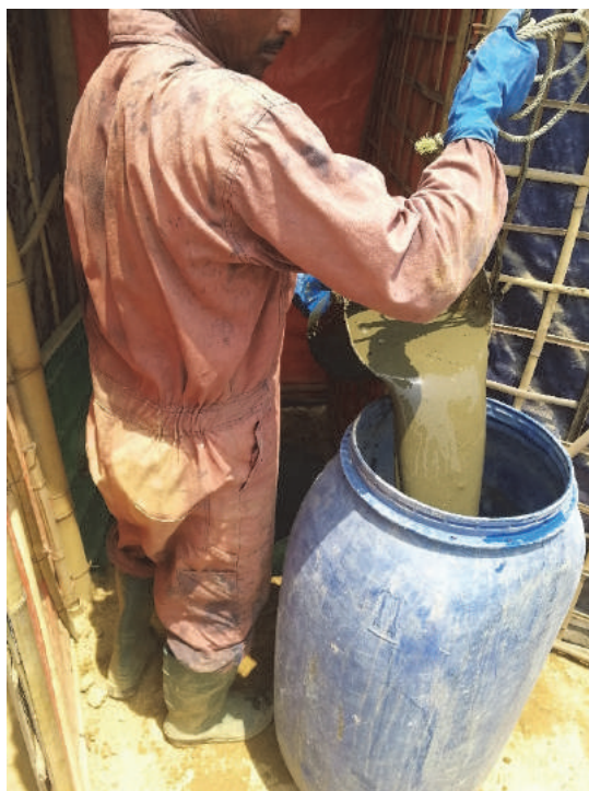
Figure 2.5.1 Manual emptying of faecal sludge with buckets and rope into barrels.
