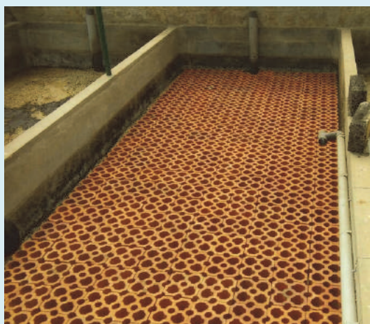
Figure 3.3.4 Mangalore tiles and their arrangement prior addition of the sand layer.
