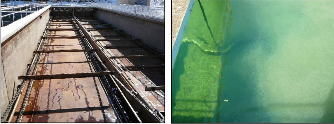
**Figure 26: Rectangular clarifier sludge removal system**
