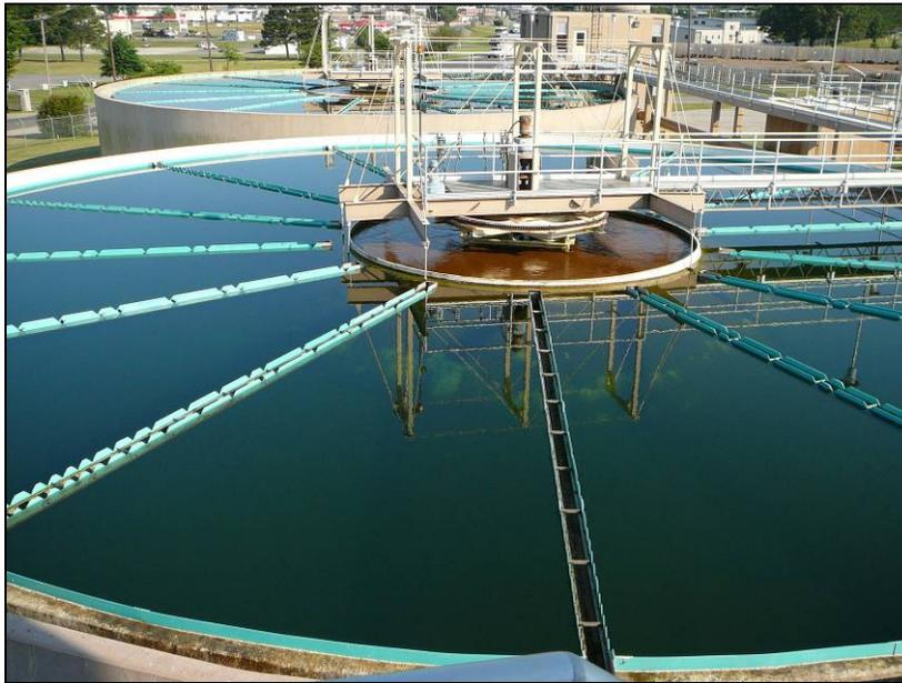
**Figure 34: Circular drinking water clarifier with radial launderers and v-notch weir plates
