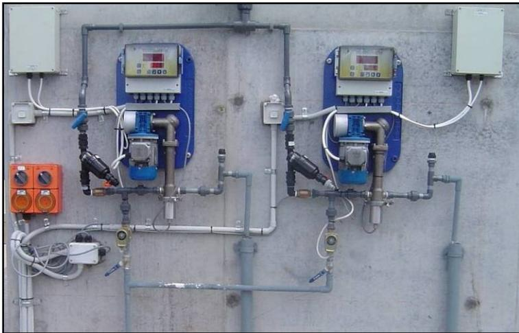
**Figure 24: Accufloc Streaming Current Monitor.**
