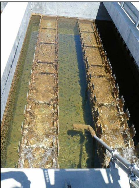
**Figure 32: Tube Settlers enhance settling**
