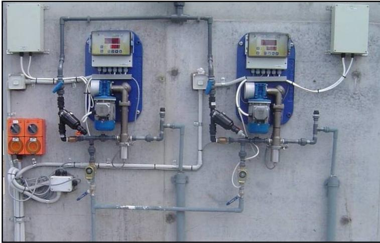
**Figure 24: Accufloc Streaming Current Monitor.**
