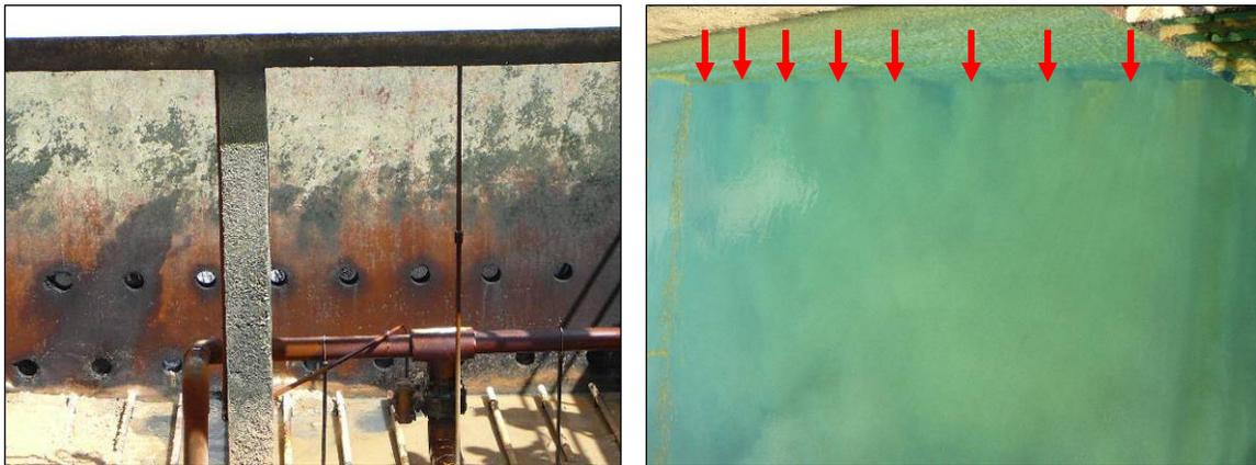
**Figure 27: Clarifier w/ perforated inlet baffle wall**
