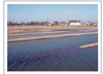
Figure 3. Man-made infiltration basins are an example of direct recharge.
