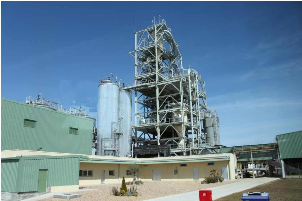
Figure 58: Second generation ethanol plant of ABENGOA in Spain (Source: Rutz D.)
