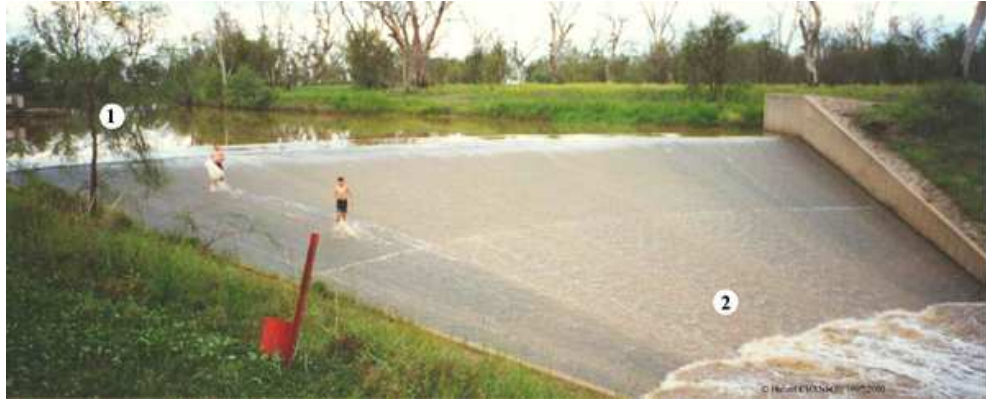
Figure 15.8: Water flowing down a weir, which is a type of rapidly varied flow. The Bernoulli principle may be applied between Points 1 and 2. [Photo ©Chanson 2000]
