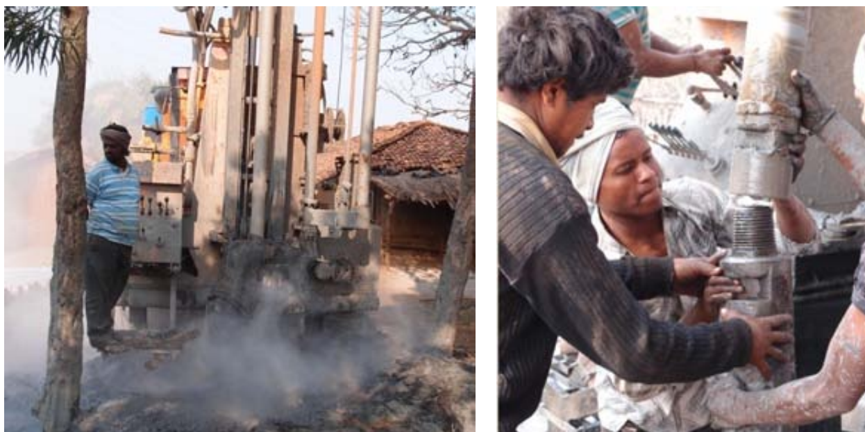
Figure 22: Drilling of new 90 m well at Lalpur disinfection pilot plant.
