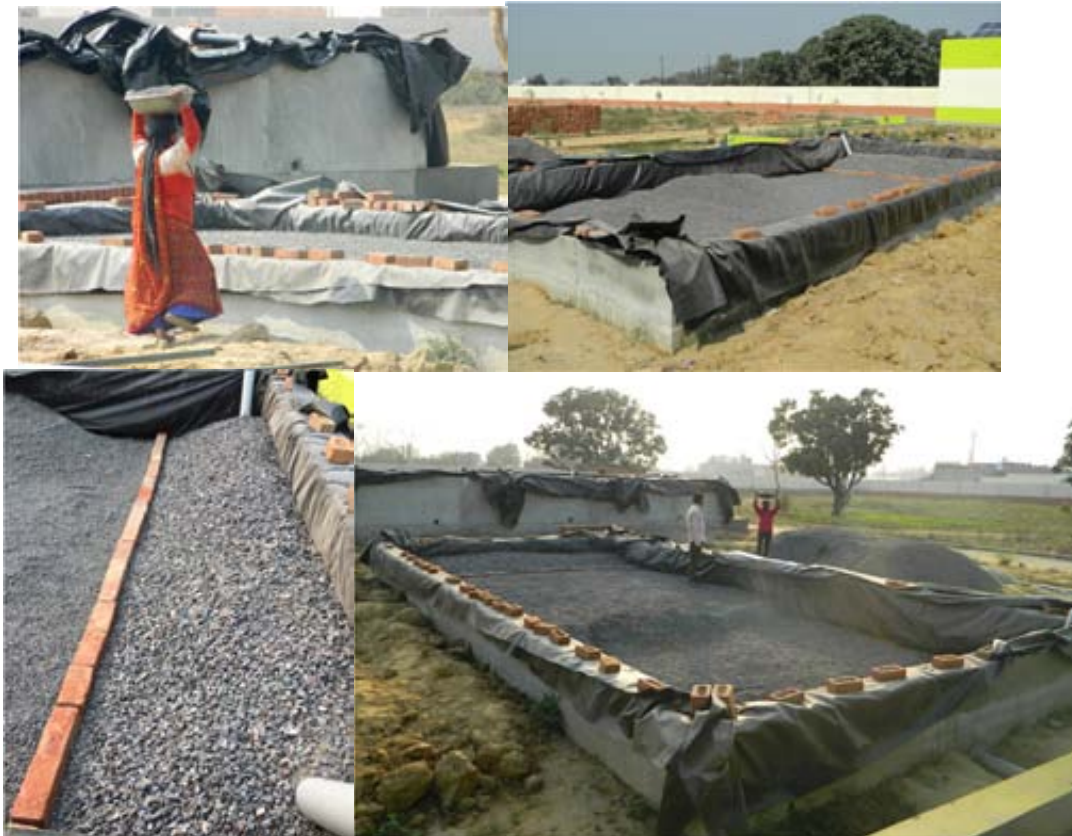
Figure 10: The horizontal flow bed during the gravel filling stage.
