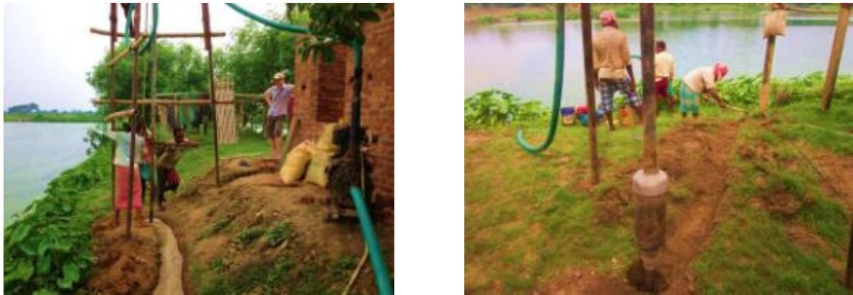
Figure 13: Drilling of bank filtration well 1 and well 2.
