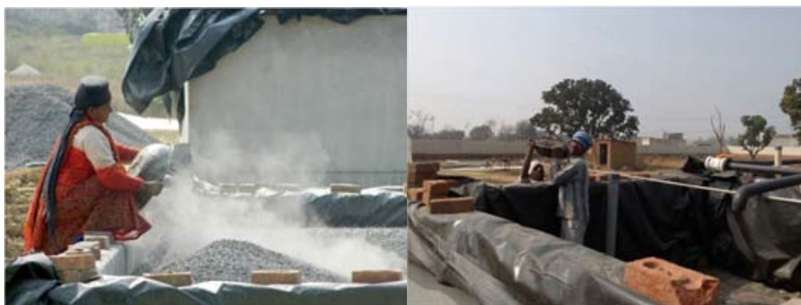
Figure 8: View of the initiation of filling of the FS VF beds.
