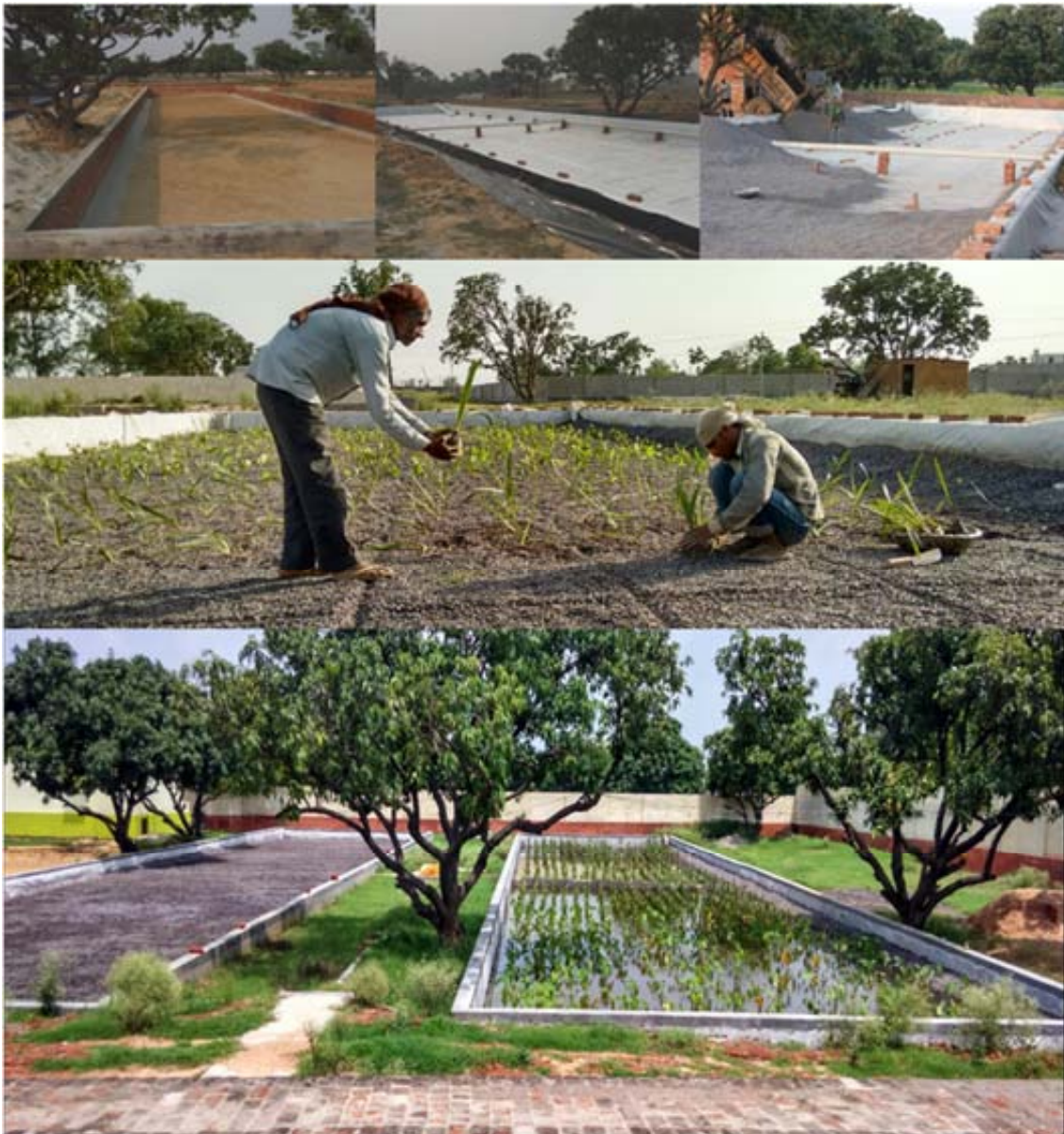
Figure 5: Horizontal constructed wetlands implementation.
