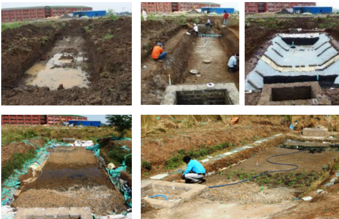
Figure 27: Construction of planted gravel bed filter at Amarkantak IGNTU site.
