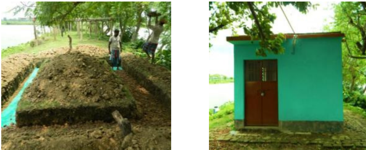
Figure 16: Finished building for disinfection systems.
