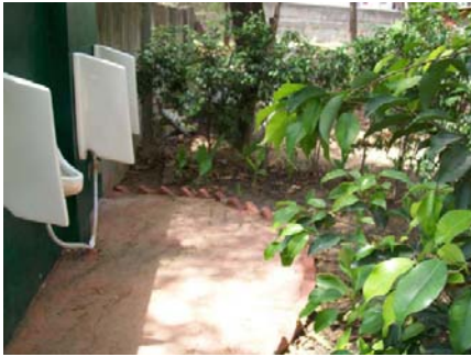
Figure11. Green urinal established at IIT Delhi (Photo: R.Sakthivel)
