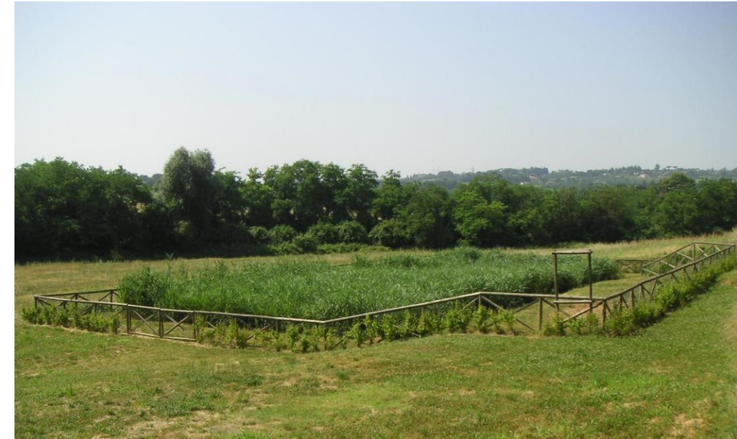
Horizontal flow system for 120 P.E. in Central Italy, operating since 2003
