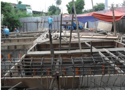
DEWATS plant for several buildings (above) and under full construction (below)
